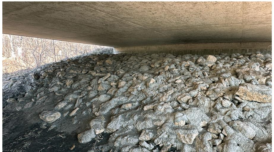
*Partially grouted revetment under a low-volume bridge*
