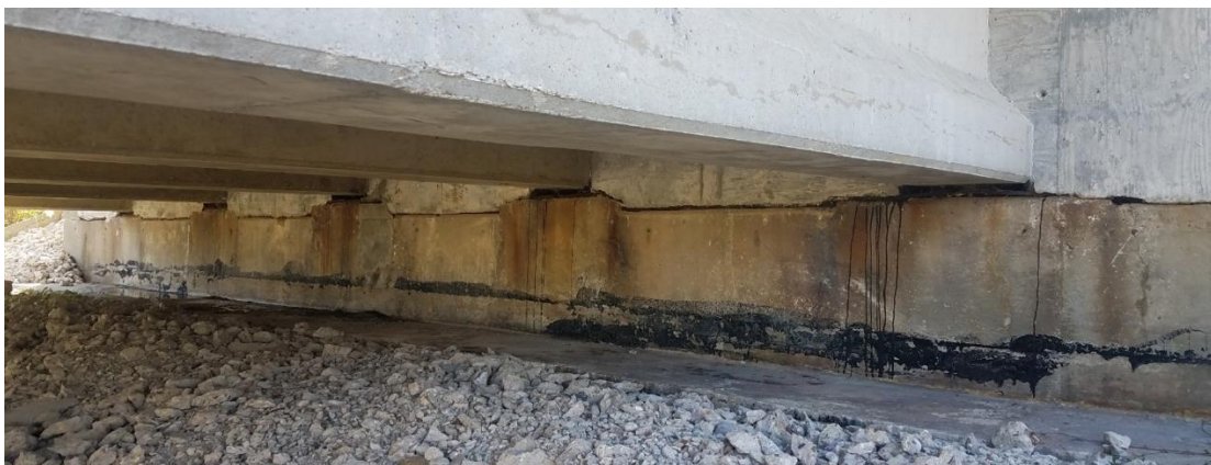
Figure 3.7. Abutment face showing the new backwall on top of the old footing
