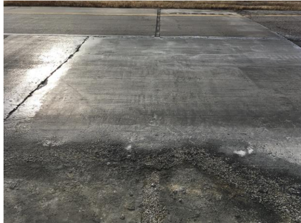
Figure 2.32. Asphalt patch
