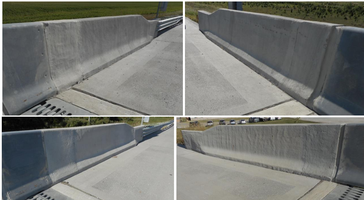
Figure 2.47. Bridge inspection photographs
