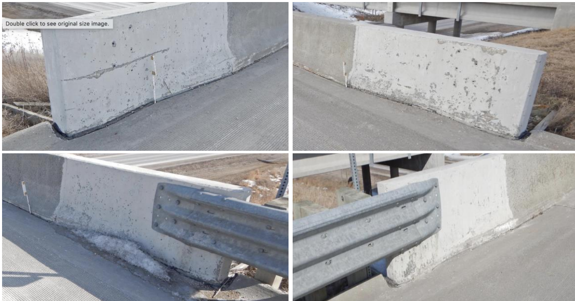
Figure 2.41. Bridge inspection photographs—barriers
