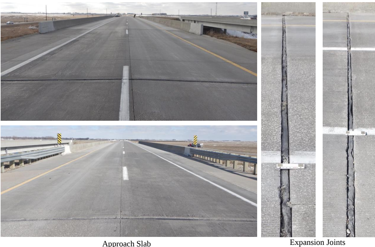
Figure 2.40. Bridge inspection photographs—approach slabs
