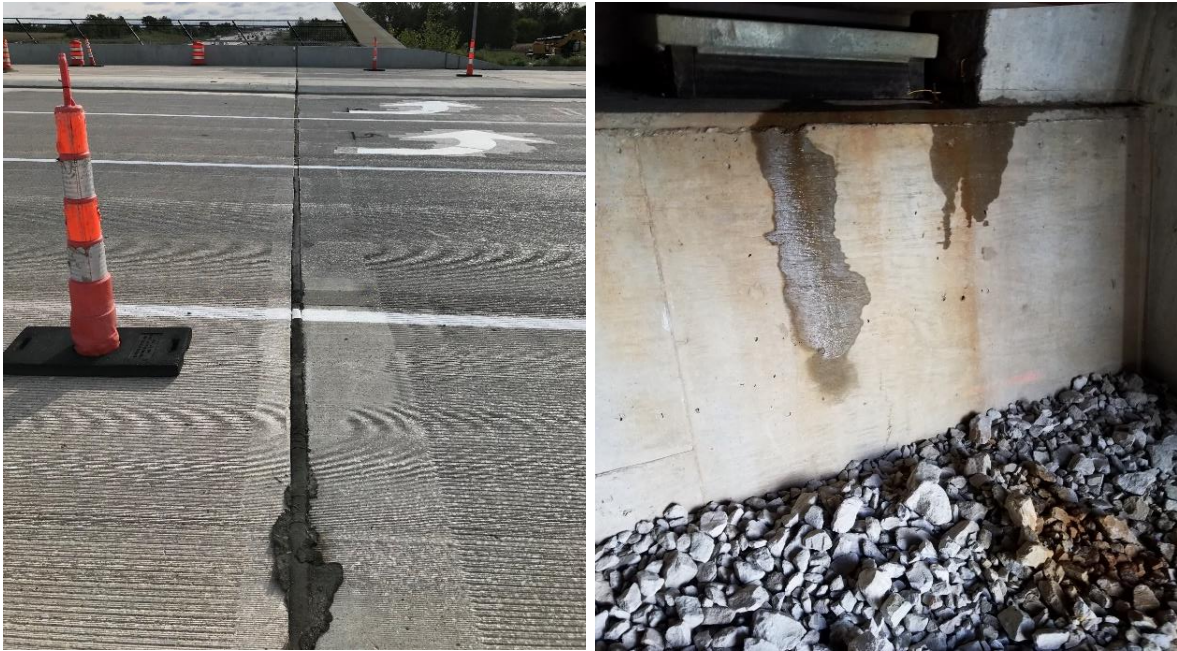
Figure 3.1. South bridge-deck-to-approach-slab joint with excess sealant (left) and water and abutment staining at the outermost girder (right)
