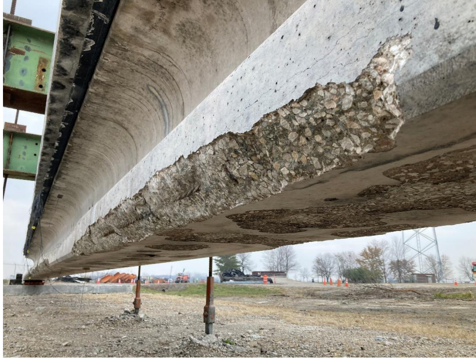
Figure 74. Bottom flange after loose concrete removal
