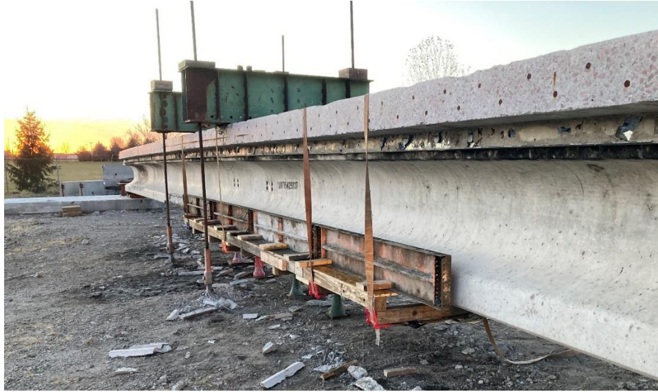
Figure 77. Steel and plywood formwork
