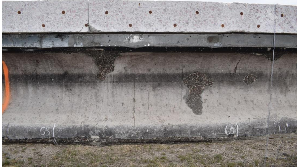
Figure 47. Web spalling on Girder E
