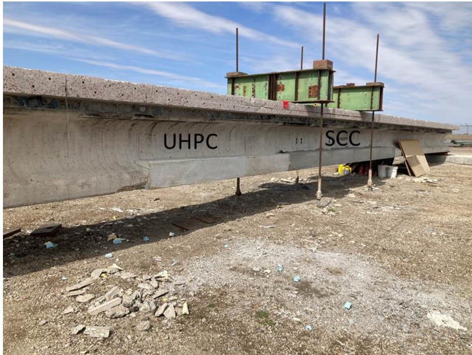
Figure 81. UHPC and SCC repair sections fully cast
