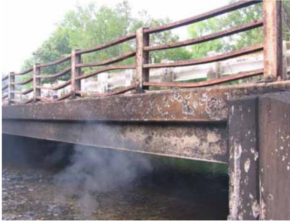
Figure 17. US 7 Bridge fascia after fire
