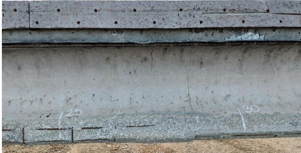
Figure 50. Exposure of steel reinforcement as a result of concrete spalling on Girder G
