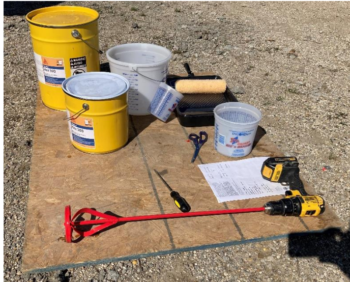
Figure 85. Preparation for mixing the FRP resin
