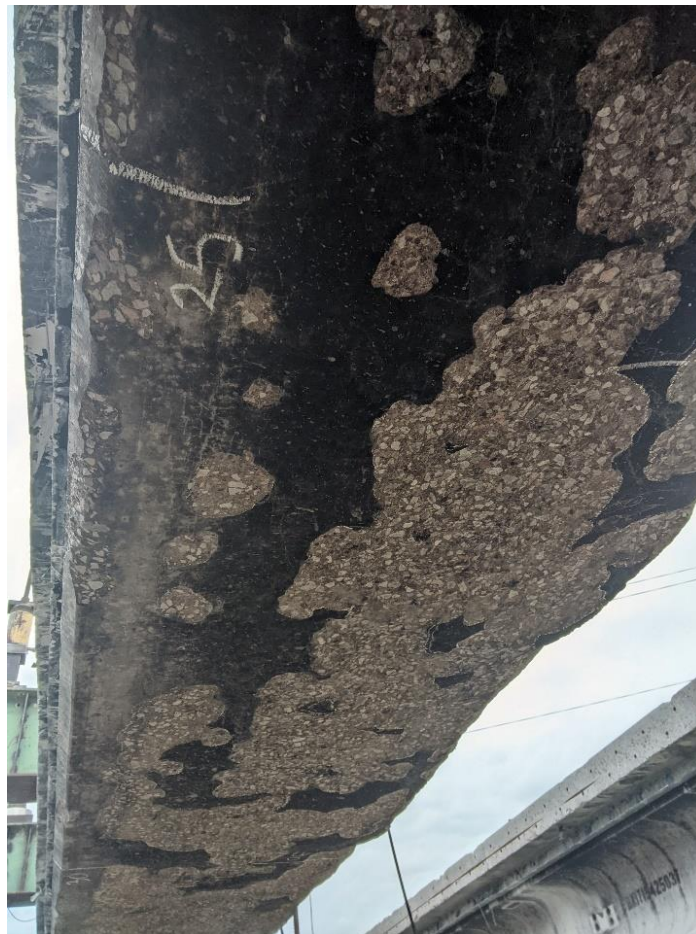
Figure 48. Bottom side spalling on Girder E
