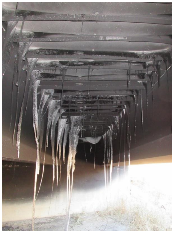
Figure 4. Melted polycarbonate stay-in-place forms
