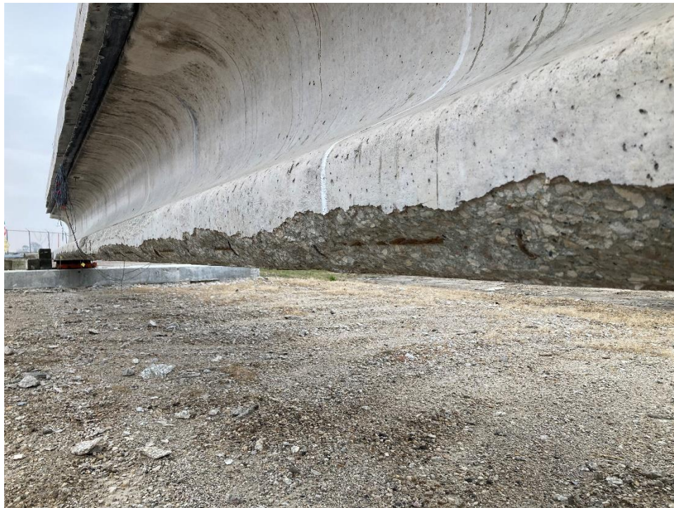
Figure 73. Removal of loose bottom flange concrete
