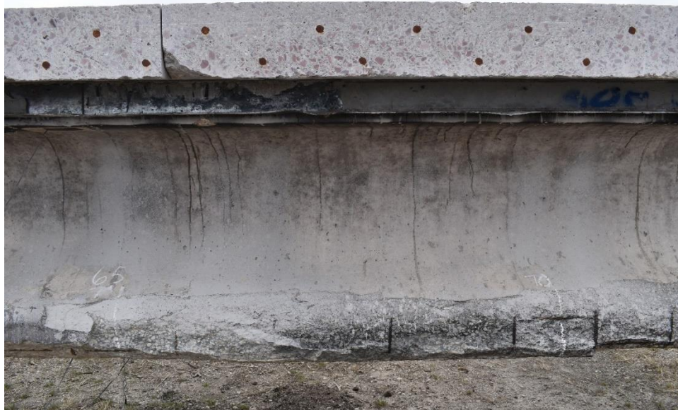
Figure 46. Bottom flange spalling on Girder E
