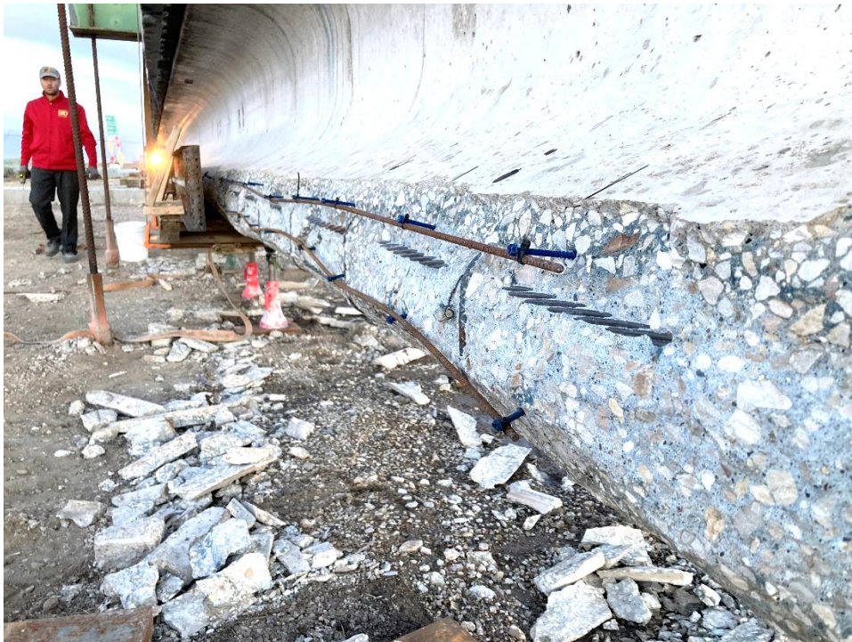
Figure 76. Tapcon concrete anchors and #3 rebar
