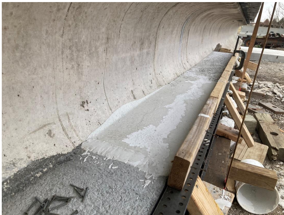
Figure 80. Placement of the UHPC section of repair
