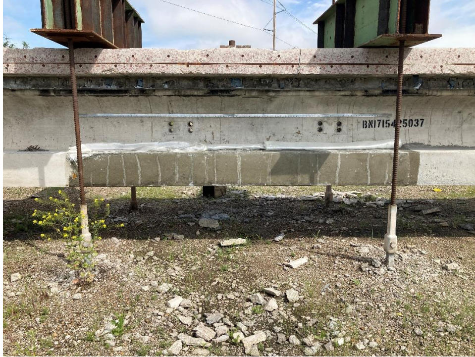
Figure 90. Vertical cracks in SCC/FRP repair section
