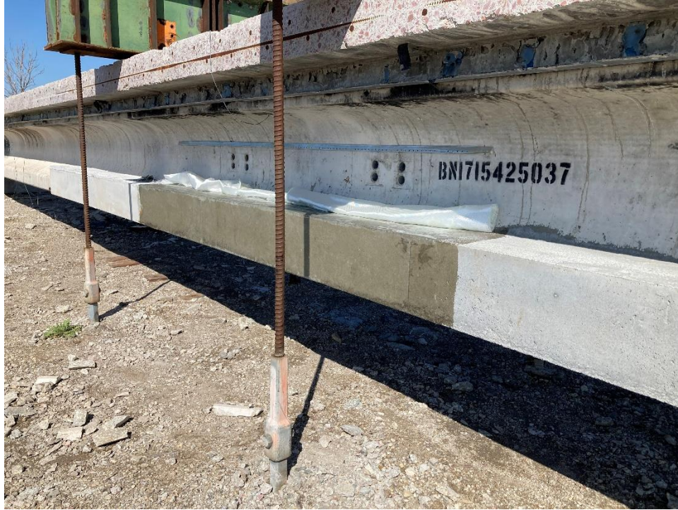
Figure 86. FRP wrap application on bottom flange repair
