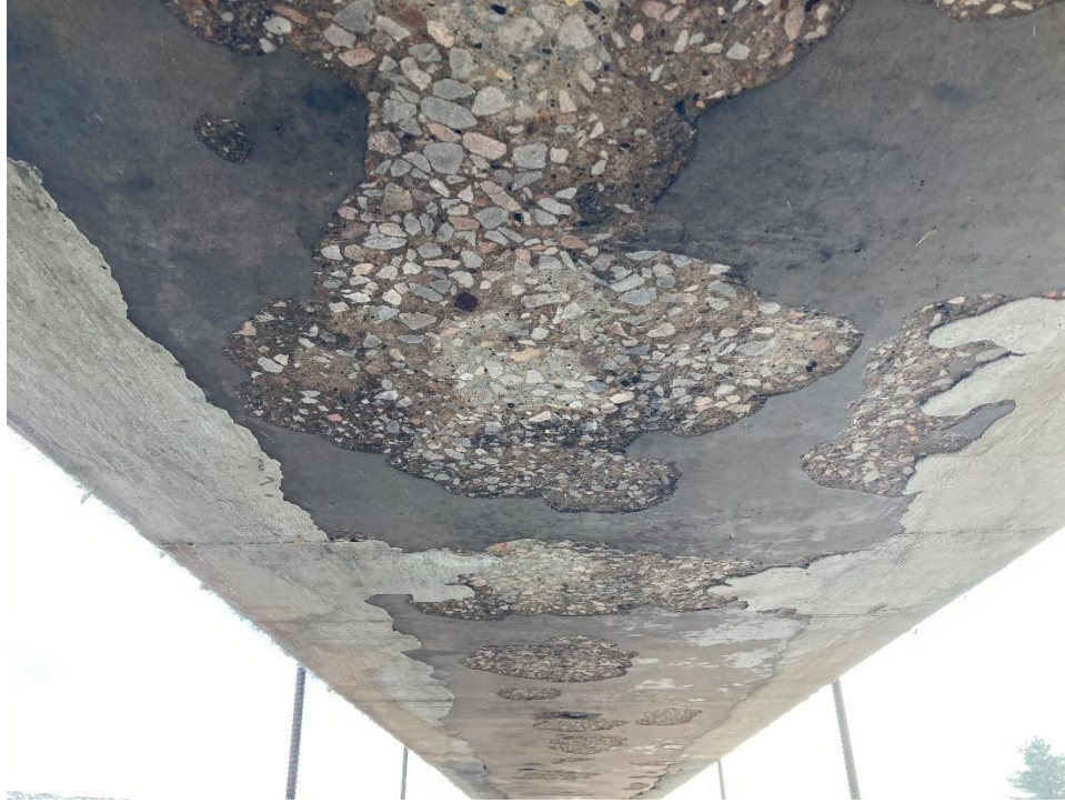
Figure 83. Bottom of girder spalls prior to repair
