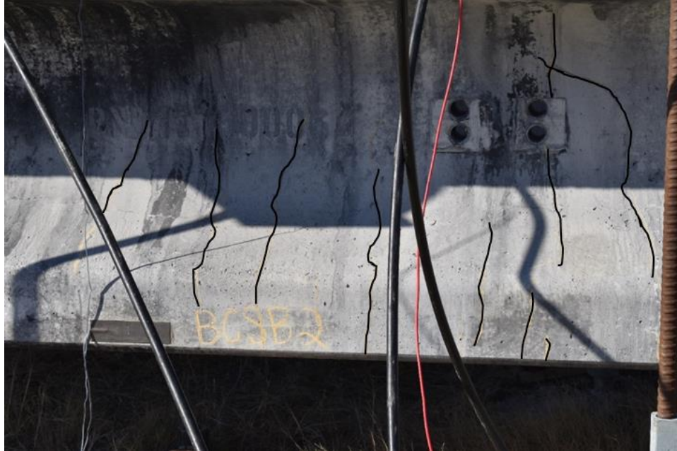
Figure 52. Crack patterns at midspan of Girder B
