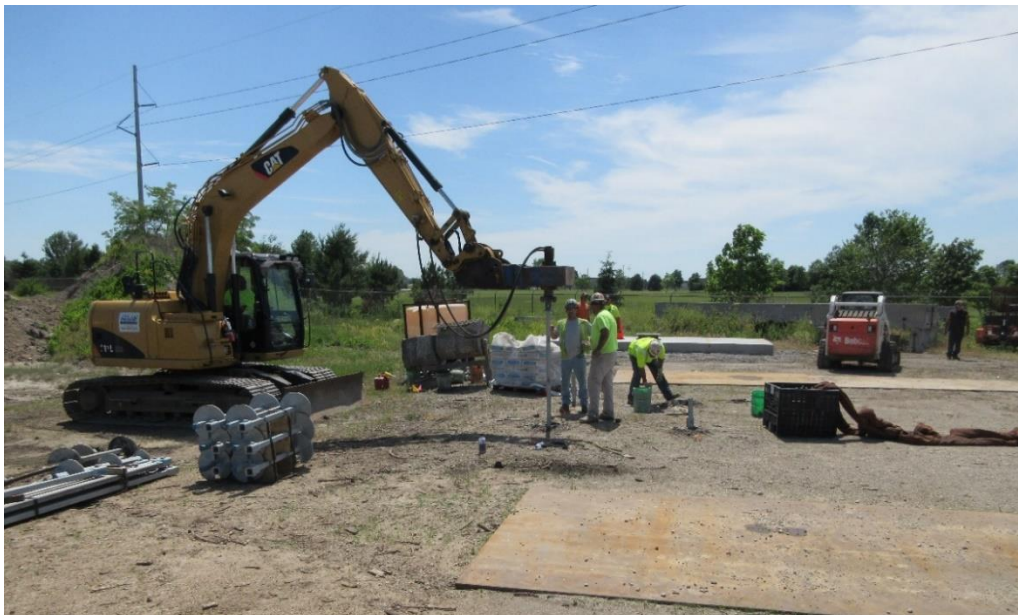
Figure 37. Installation of helical piles
