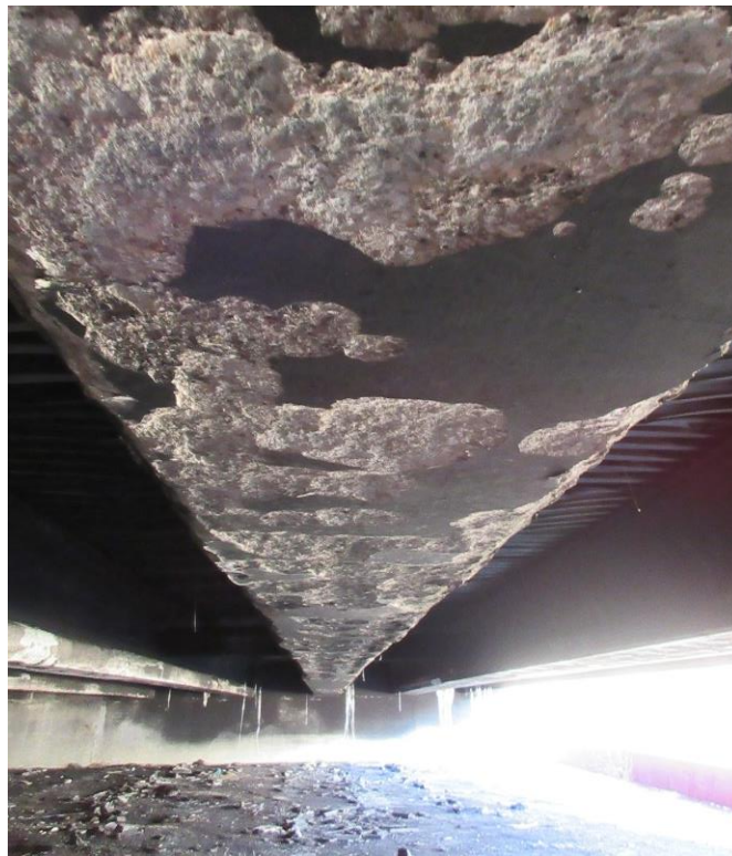
Figure 2. Concrete spalling on concrete girder
