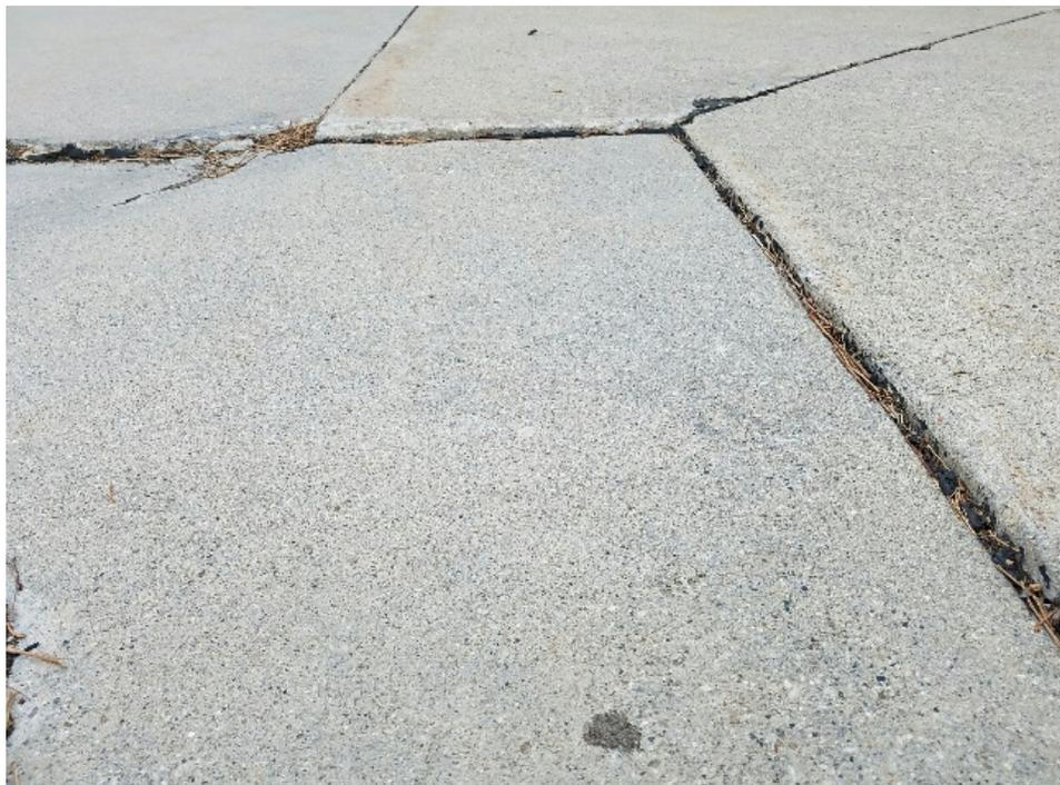
**h. Settlement due to consolidation of the subgrade soil without significant traffic loading**
