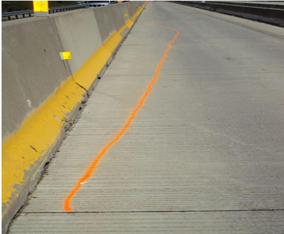
**e. Longitudinal crack along centerline joint with possible late sawing**
