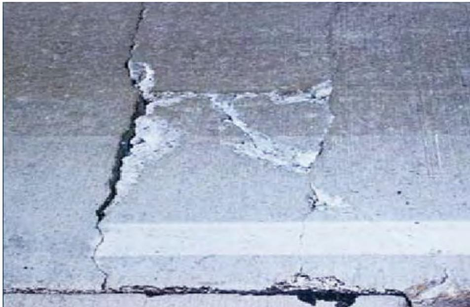
**d. High severity punchout in CRCP**
