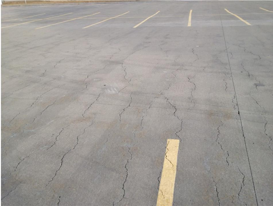
**b. Plastic shrinkage cracking**
