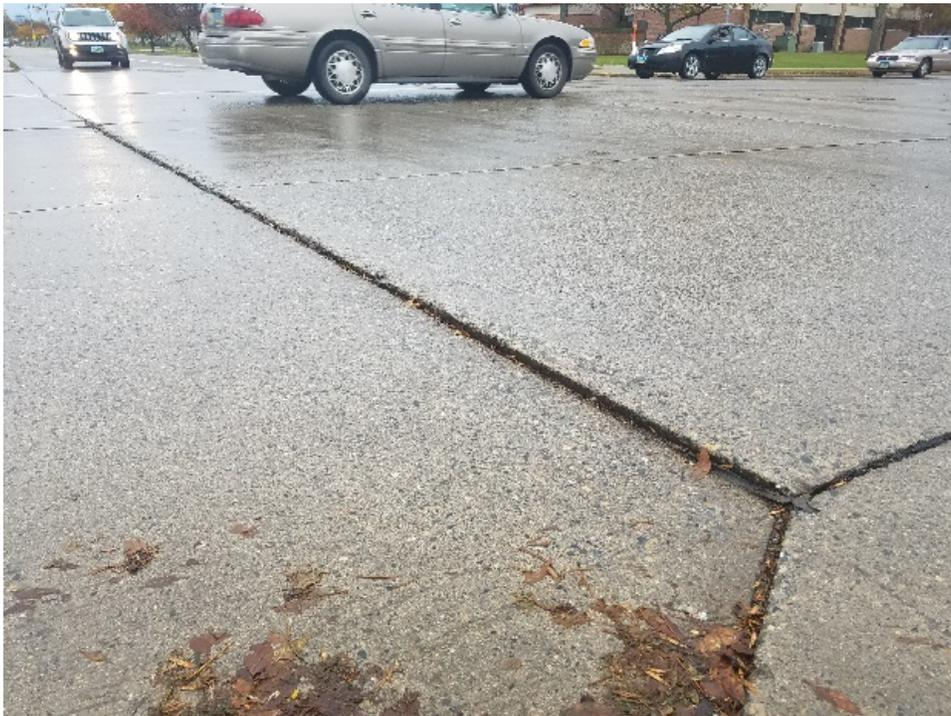
**f. Settlement due to subgrade soil movement under traffic**
