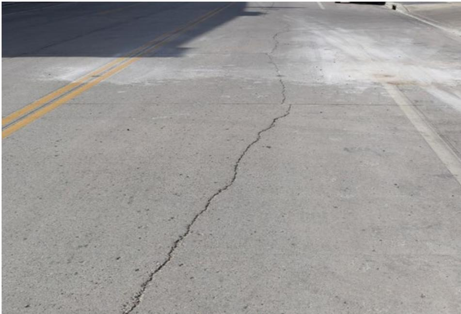
**b. Cracking due to trench backfill settlement**
