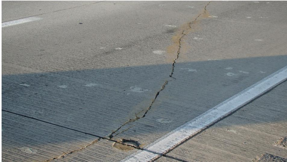
**d. Longitudinal crack over dowels at JPCP transverse joint**
