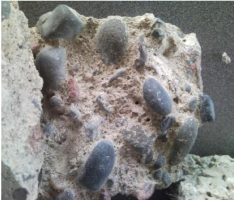
**b. Loss of the damaged paste over time, leaving exposed aggregate**
