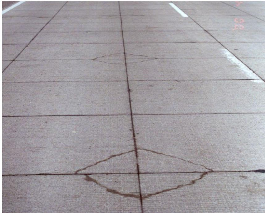
**a. Corner cracking at interior locations (early stages)**
