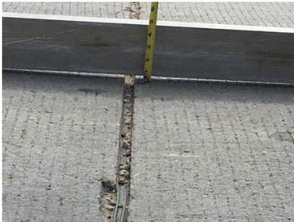
**b. Downward slab curvature visible at a transverse joint under straight edge**
