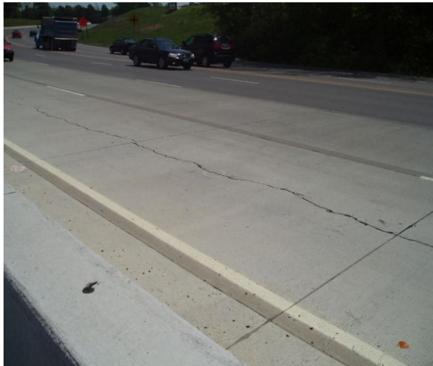
**a. Longitudinal crack (with 0.2 inch faulting) on JPCP**
