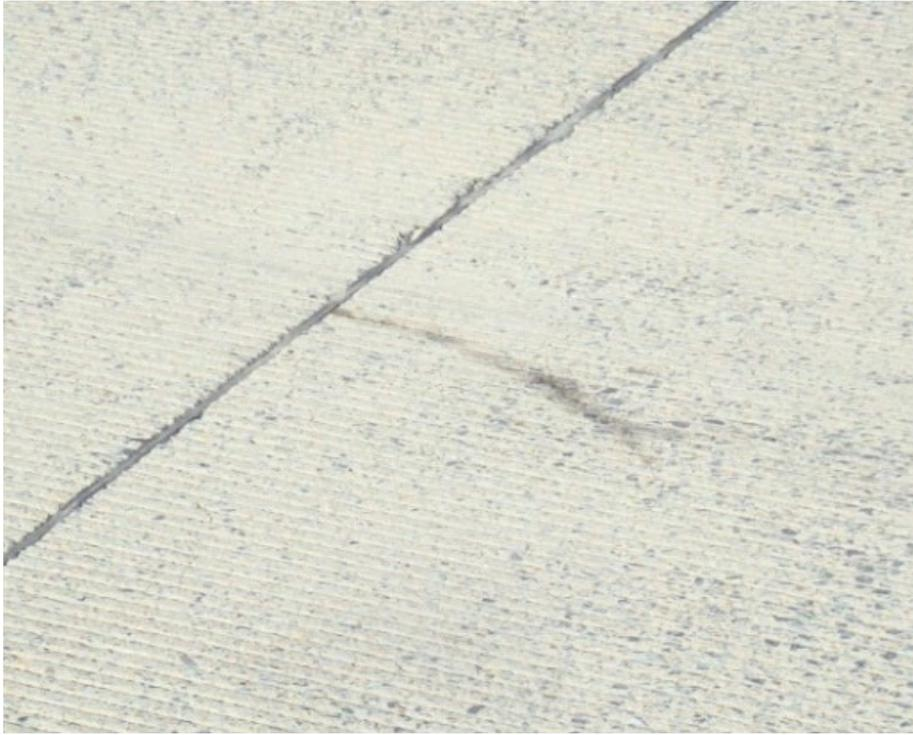
**a. Longitudinal crack, possibly due to reflection or joint restraint (improper sawing)**
