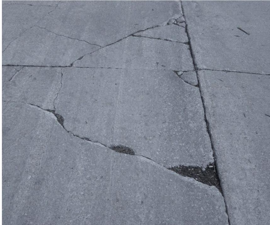
**c. High-severity interior corner breaks**
