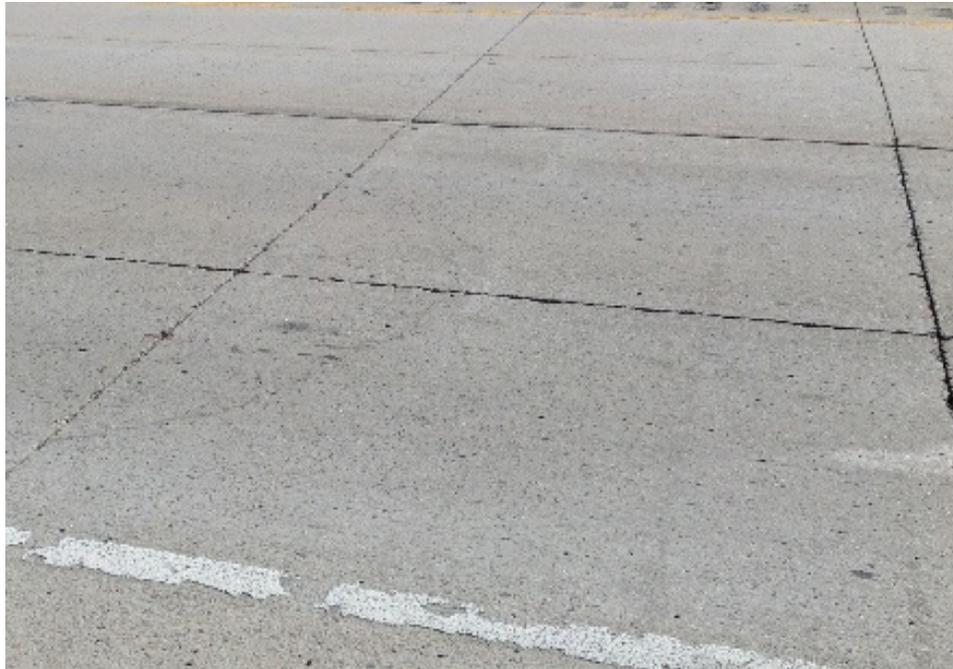
**c. Corner cracking of UBCOC**
