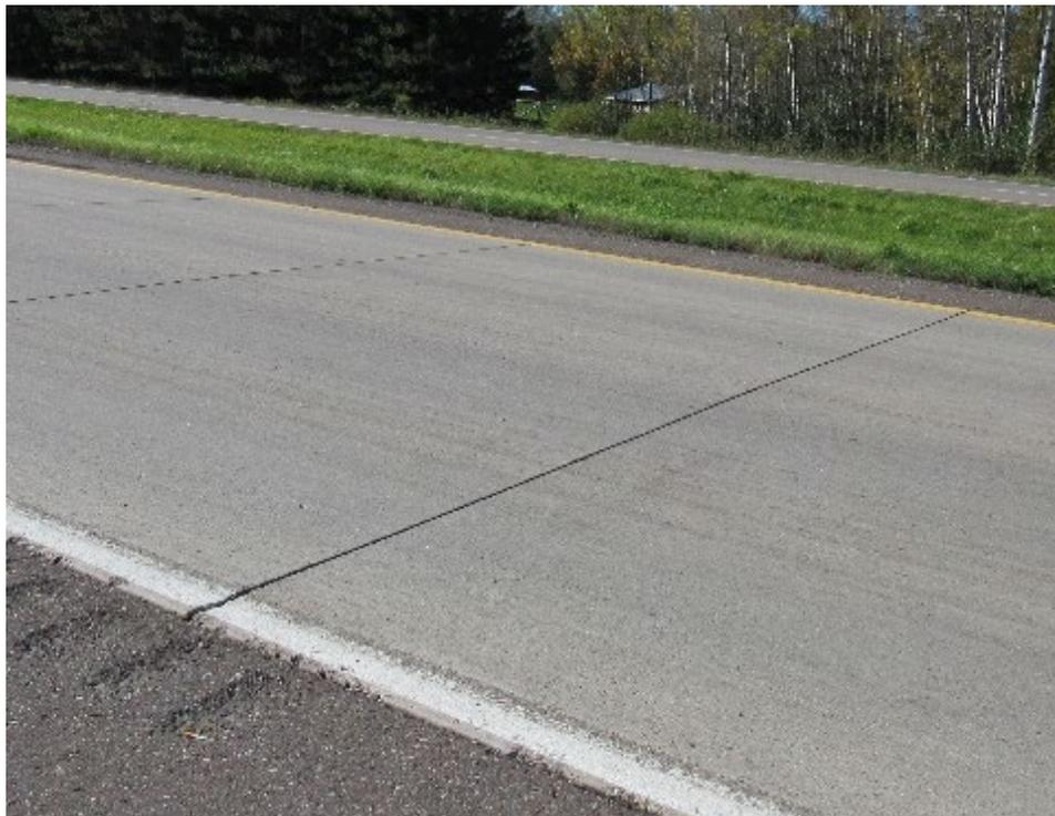
**h. Transverse joint faulting of UBCOC**
