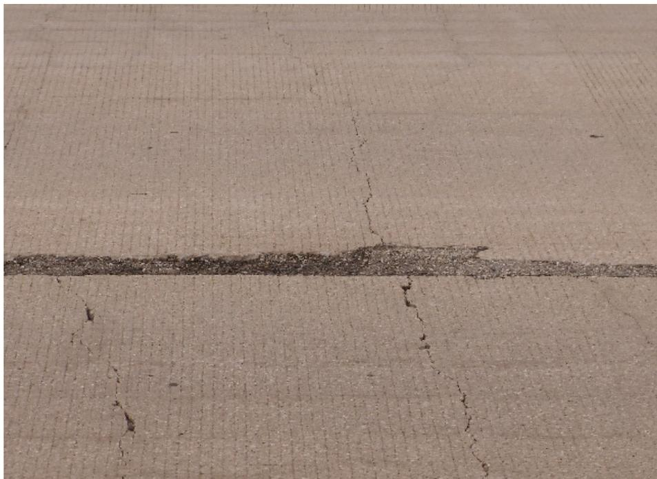
**b. Moderate severity irregular transverse cracking in CRCP**
