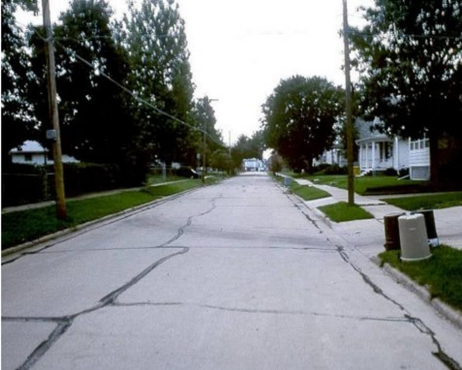
**f. Reflective transverse and longitudinal cracking due to no placement of overlay joints**
