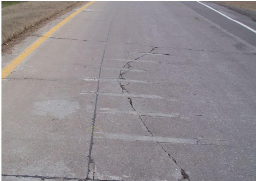
b. Slot-stitched longitudinal crack
