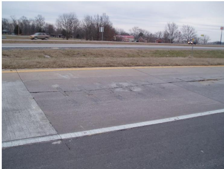
**b. Longitudinal cracking (with slot stitching) in wide ramp lane in Missouri**
