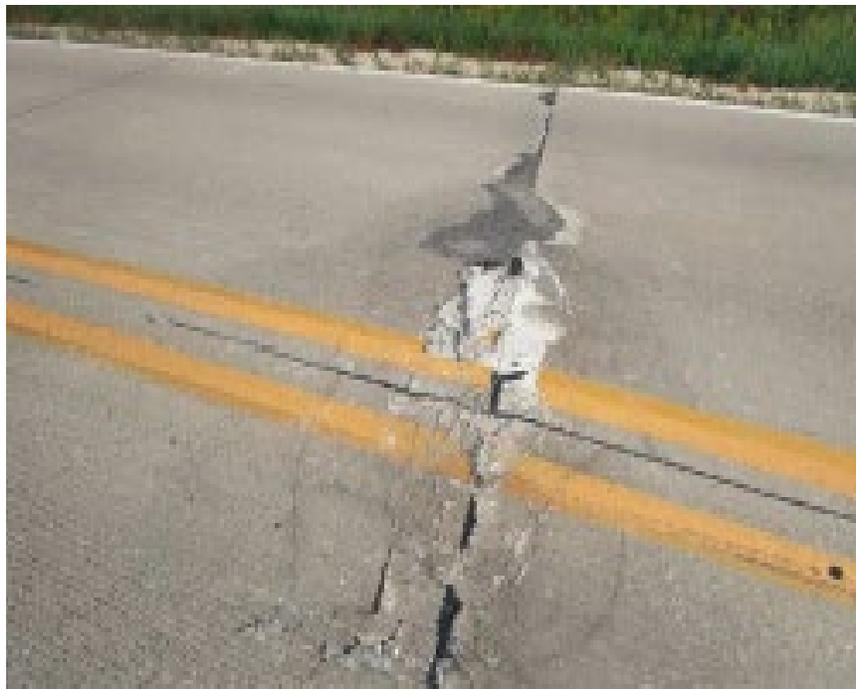
**1. Compression at transverse joint due to slab expansion and adjacent joints not opening**
