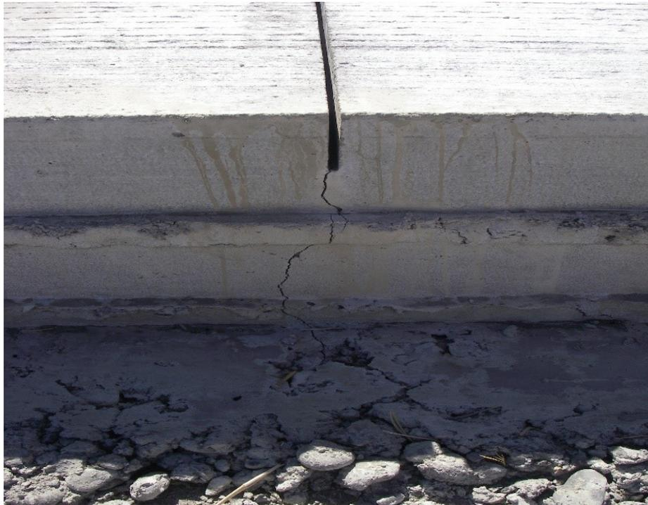
a. Proper weakened plane saw cut and induced crack
