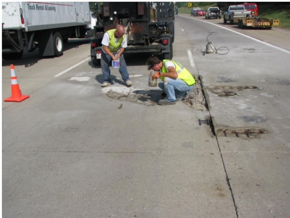
**e. Delamination due to steel mesh located near the surface**
