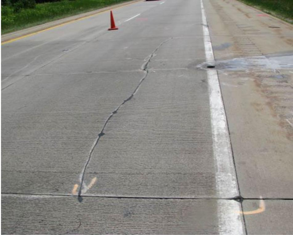
**e. Longitudinal crack due to overlay fatigue after debonding**
