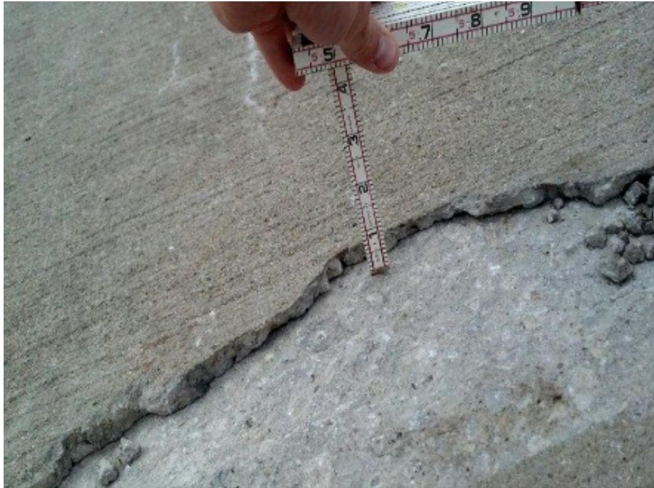
**b. Close-up view of delamination in the same location is Figure 3.1a**
