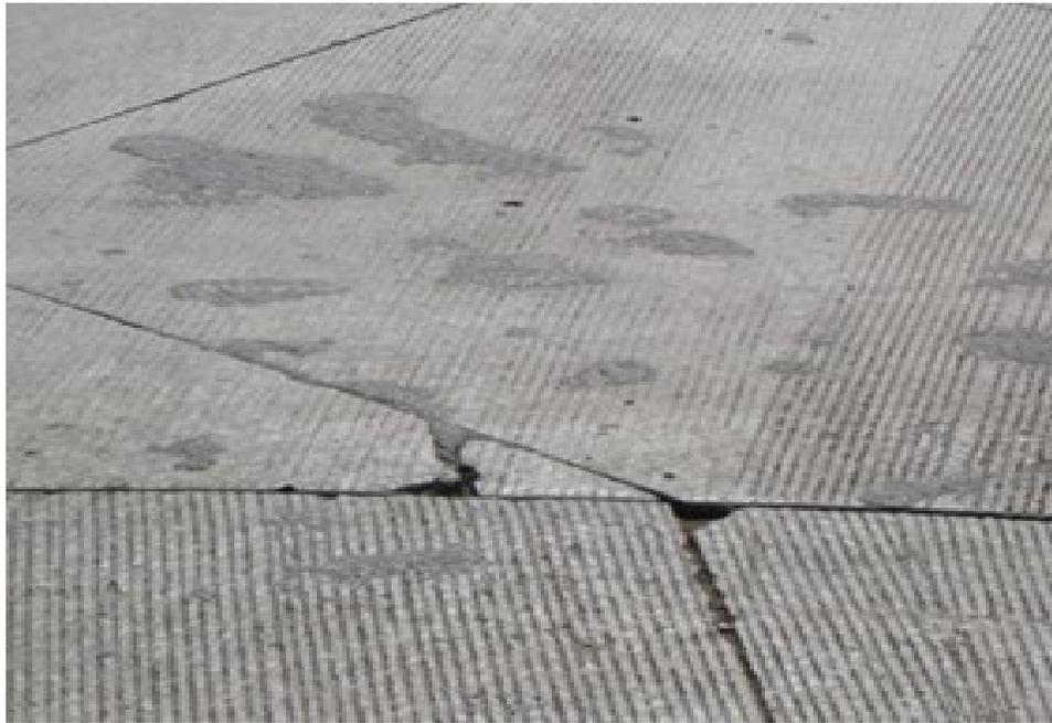
**a. Cracking due to poor joint layout**
