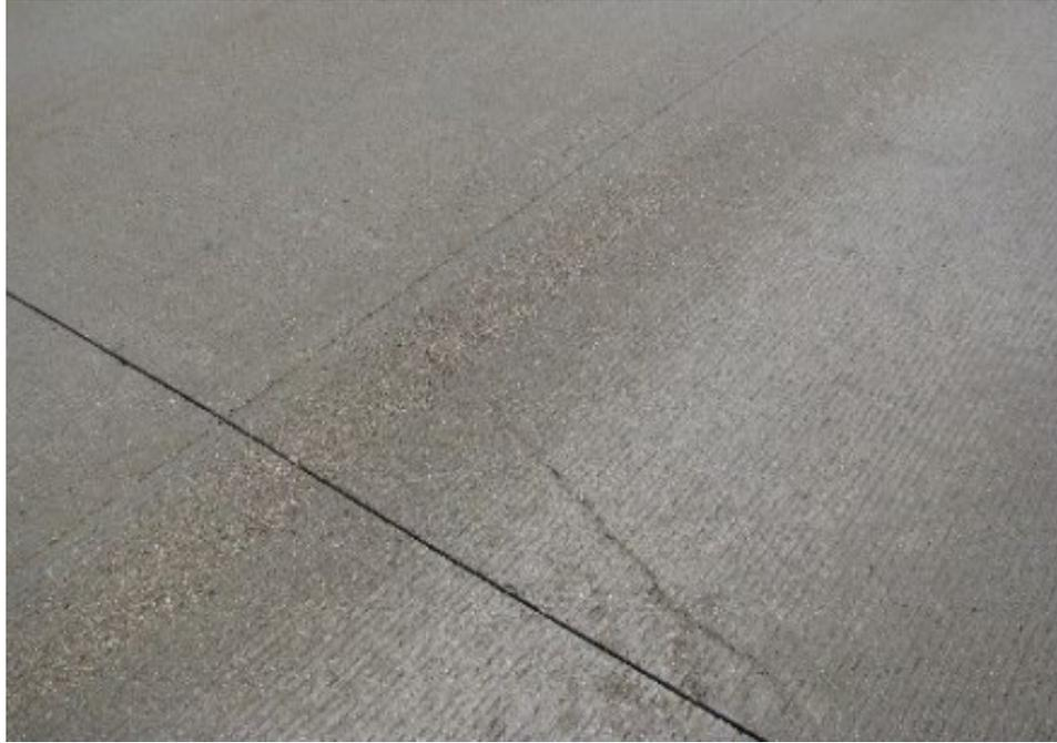
**e. Irregular reflective cracking of UBCOC**
