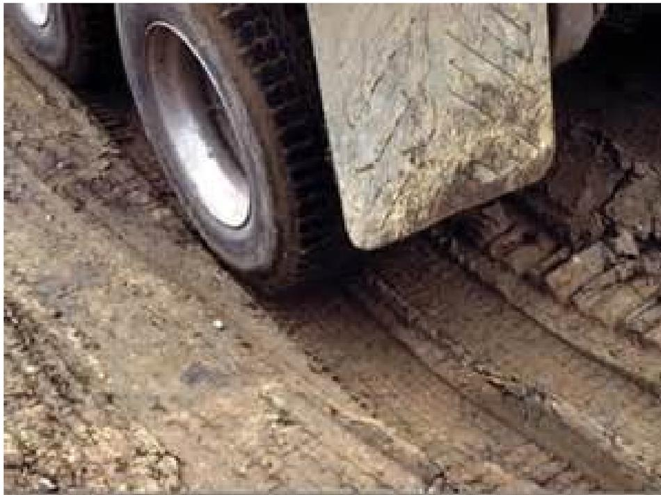
**c. Proof rolling used to determine weak areas in the subgrade and/or base/subbase**
