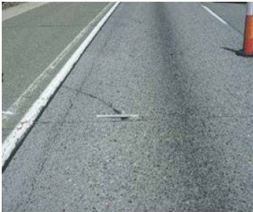
**b. Moderate-severity corner crack**
