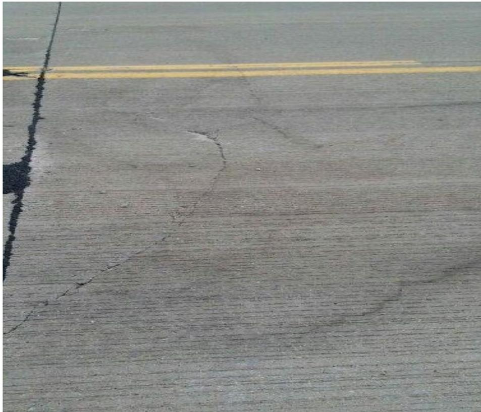
**c. Delamination and resultant cracking adjacent to transverse joint**
