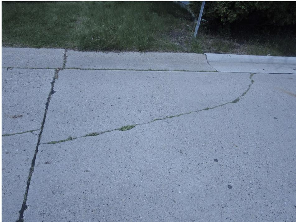
**d. Medium-severity corner crack**
