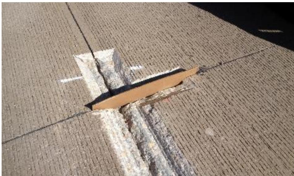
**a. Milled joints for removal of spalling for PDR**
