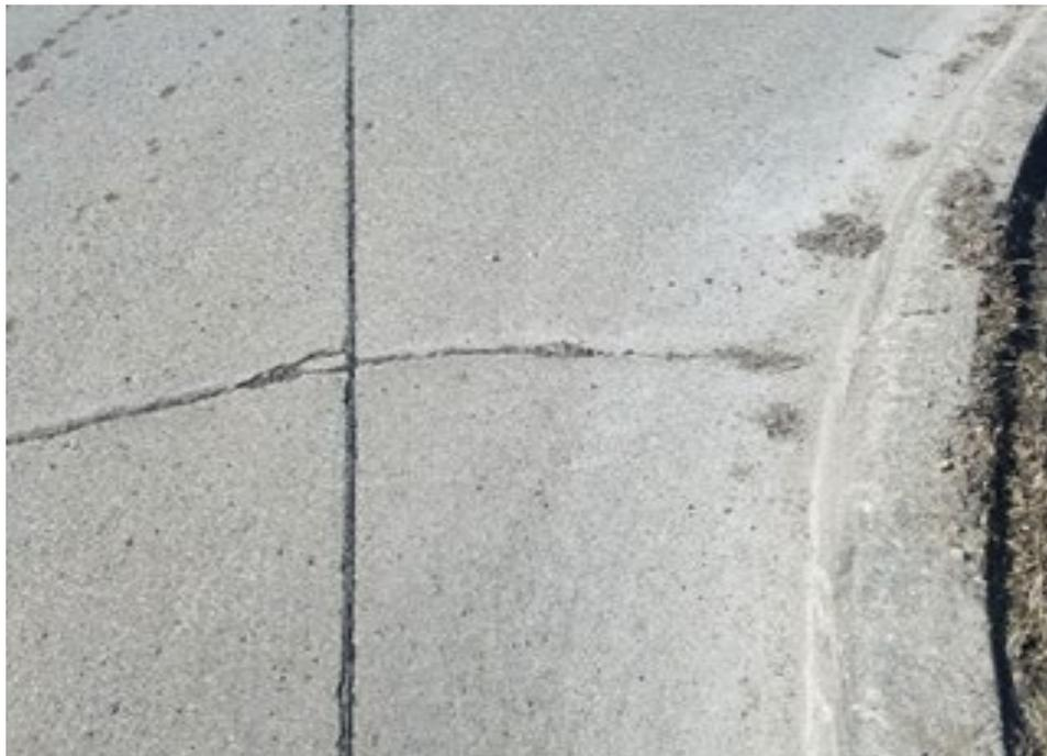
**b. Cracking caused by lack of curb saw cut**
