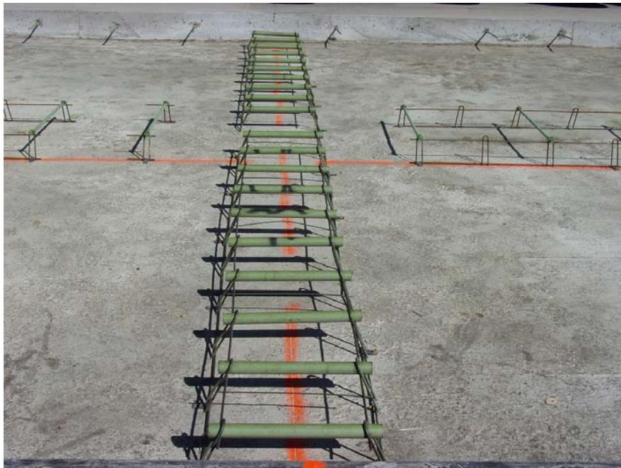
**a. Dowel bar baskets for a transverse joint and tie bar baskets for a longitudinal joint**
