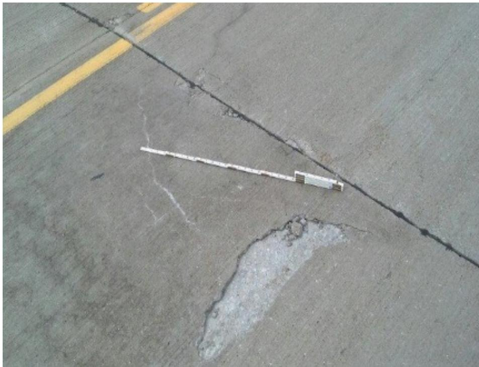
**a. Localized delamination in a conventional concrete pavement**
