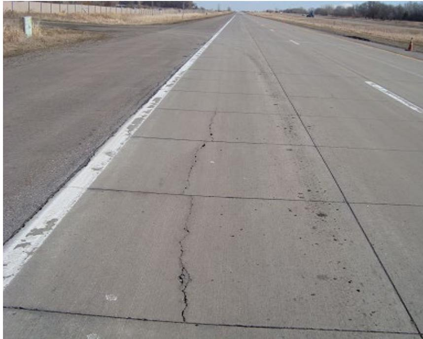
**h. Longitudinal cracking in wheel path**
