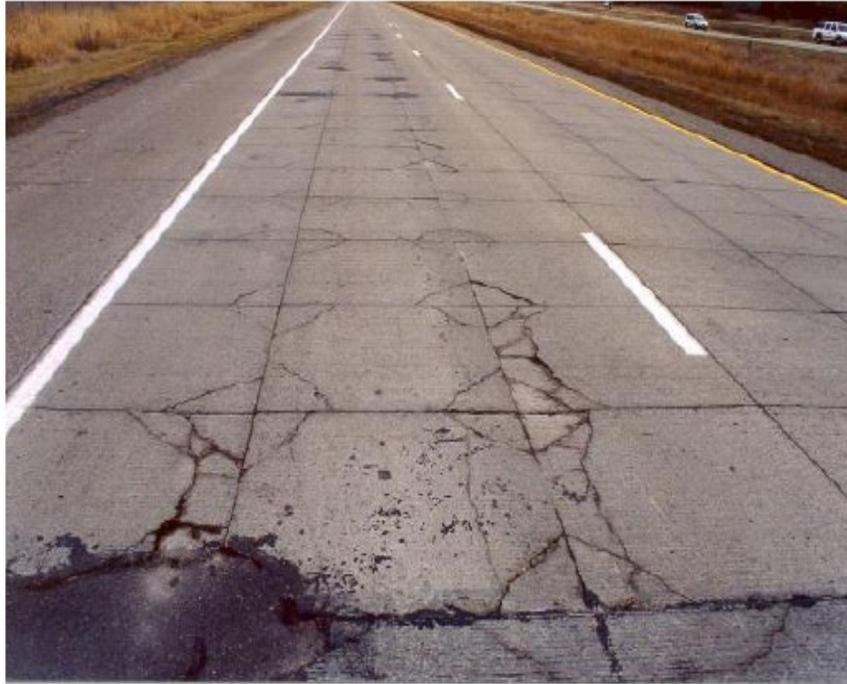
**b. Corner cracking at interior locations (late stages), leading to development of shattered panels**
