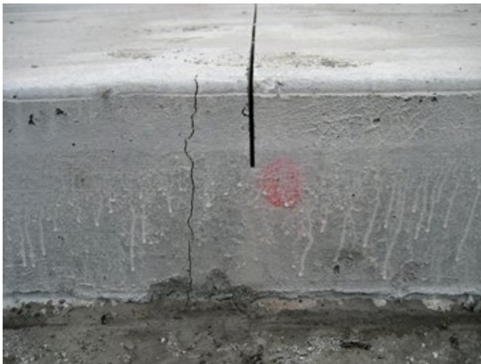
**b. Slab cracking occurring parallel to weakened-plane saw cut, possibly due to late sawing or inadequate saw cut depth**
