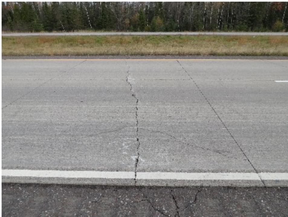
**d. Transverse reflective cracking of UBCOC**
