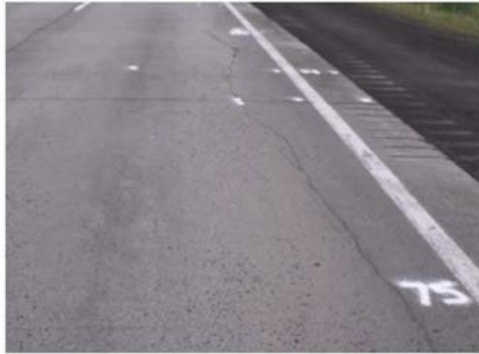
**a. Longitudinal cracking in an 8-inch pavement with a 14-foot lane width in Washington**
