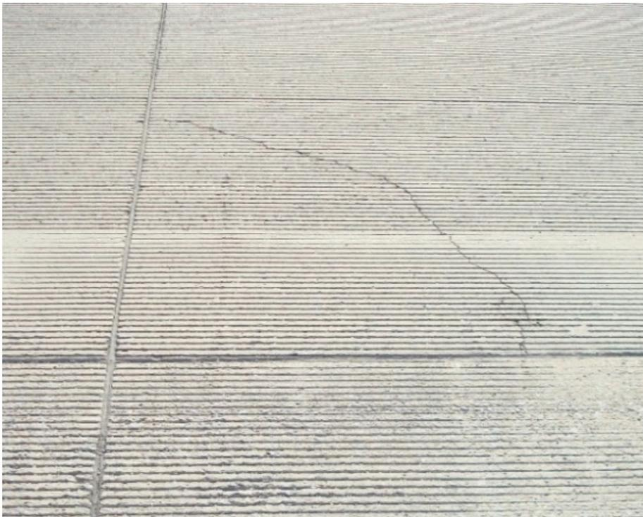
**b. Corner crack in overlay due to debonding**
