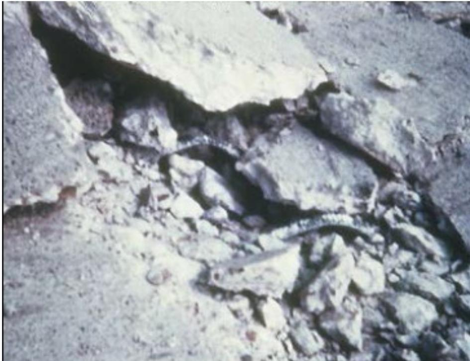
**c. Blowup in CRCP showing exposed steel**
