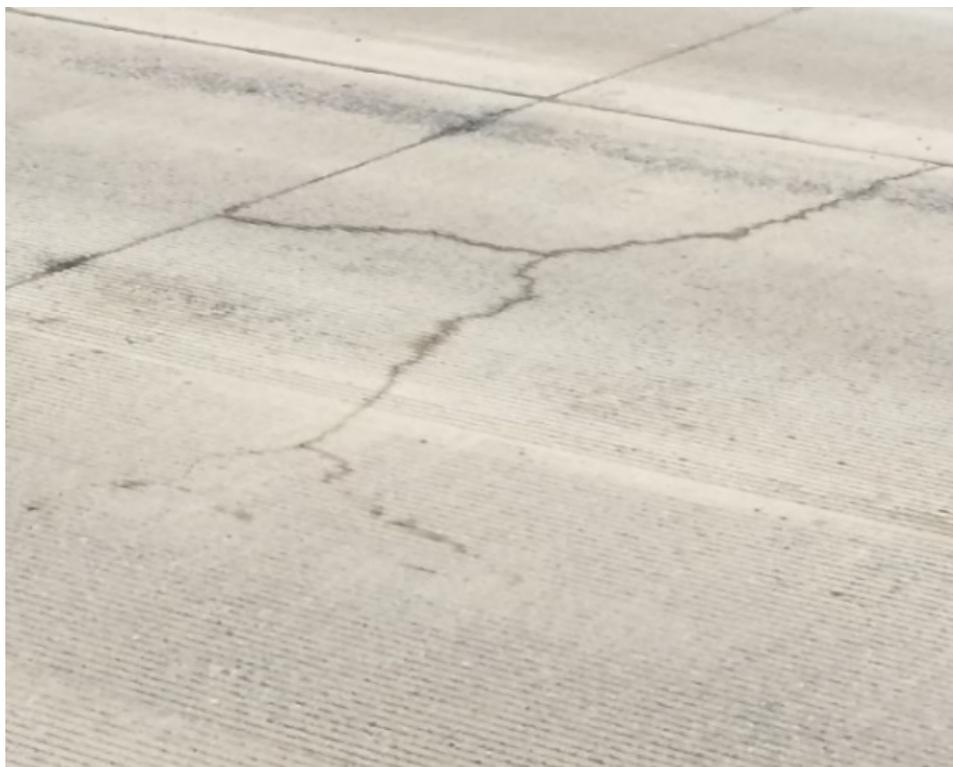
**d. Multiple panel cracks near panel end due to debonding**
