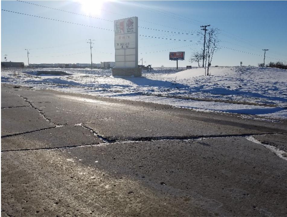
**e. High severity cracking due to frost heave of the subgrade soil**
