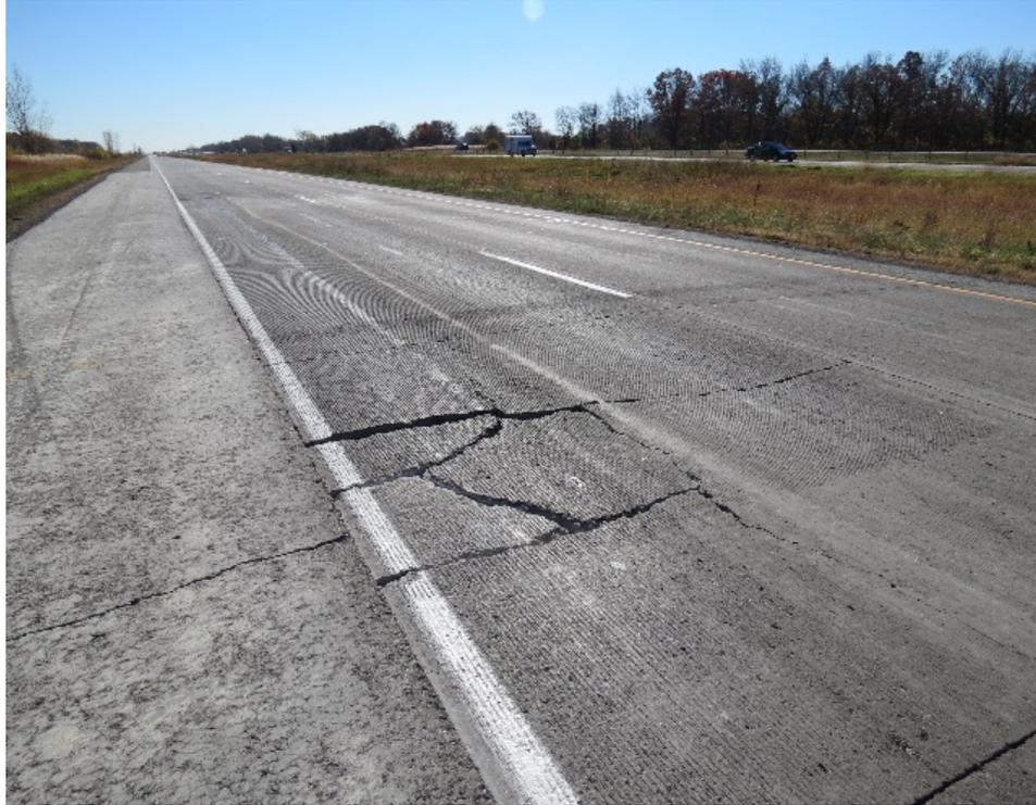
**g. High severity cracking due to settlement and loss of support**
