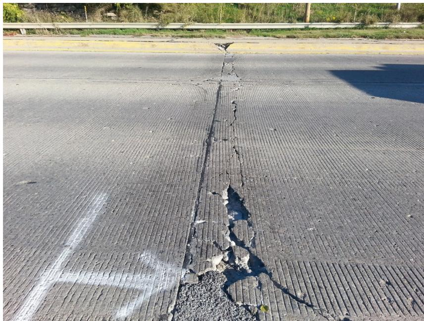
**c. Saturated joint with unsound aggregate**
