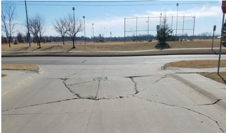
**c. Pavement settlement adjacent to a rigid structure that has not settled**
