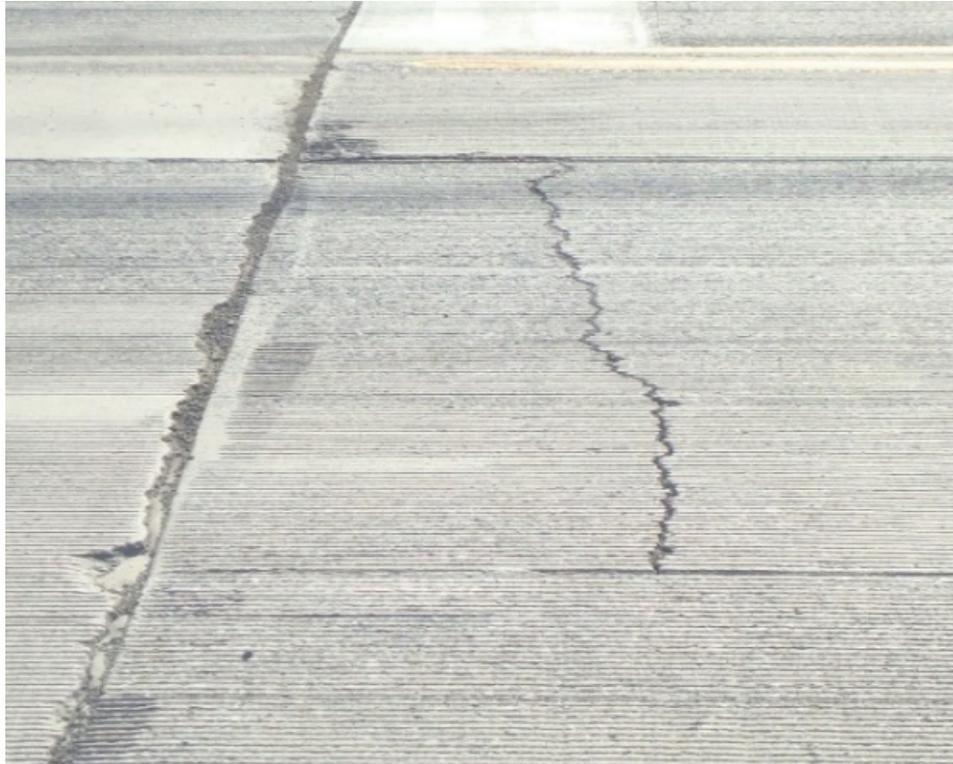
**c. Reflective crack over unrepaired transverse crack near transition**
