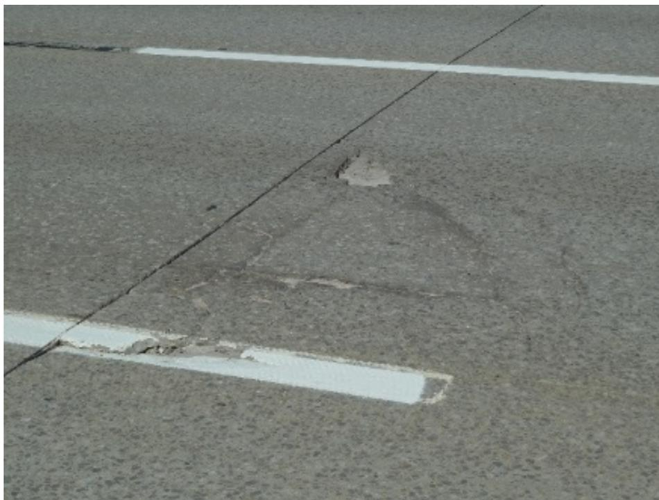
**f. Typical pattern of delamination prior to surface loss**
