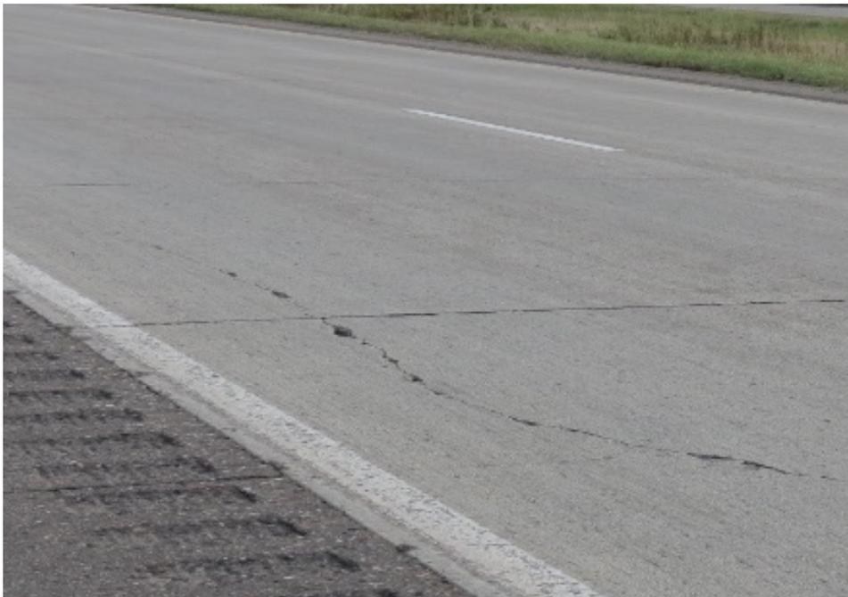
**b. Longitudinal cracking in wheel path in UBCOC**
