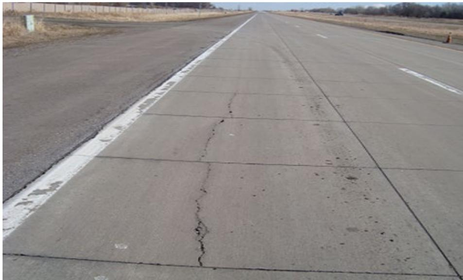
**b. Longitudinal cracking in wheel path**
