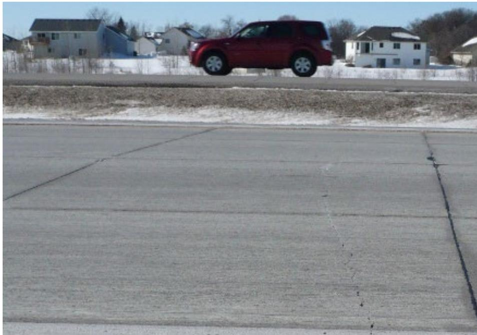
**f. Mid-panel cracking of UBCOC**
