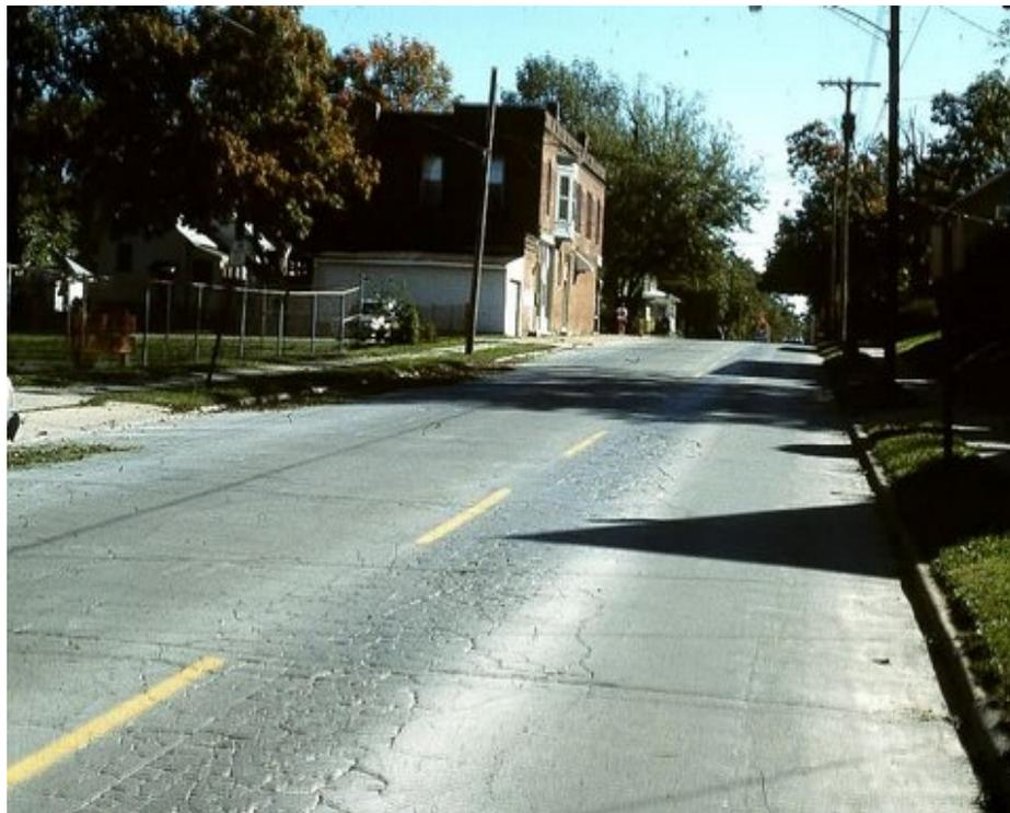
**h. Longitudinal wheel path cracking due to debonding and fatigue cracking of overlay**
