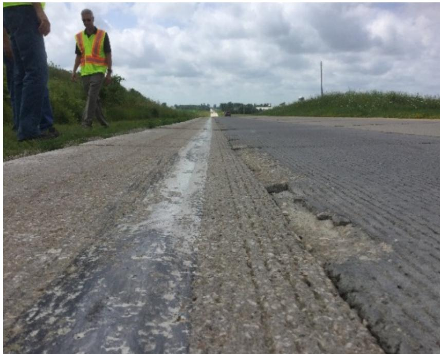
**k. Longitudinal lane-shoulder joint spall due to shoulder heave**
