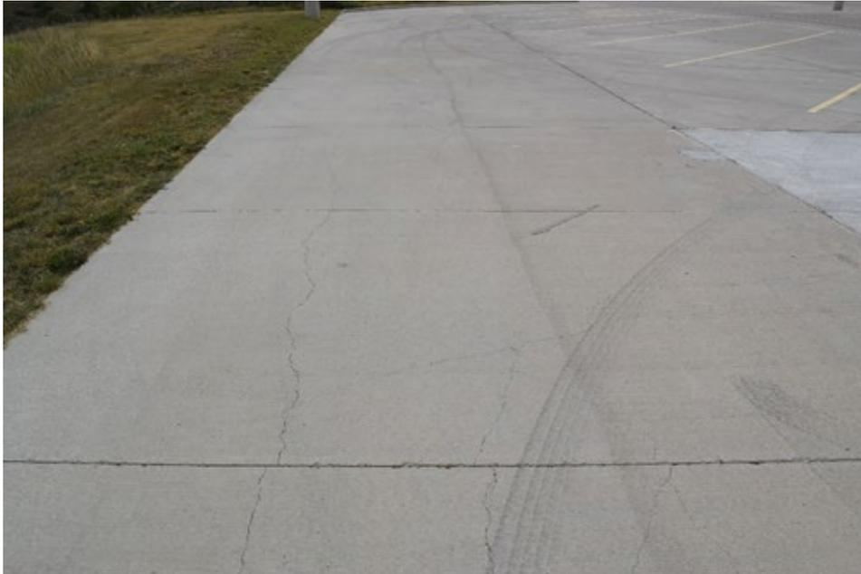
**a. Settlement due to moisture-related subgrade soil movement**
