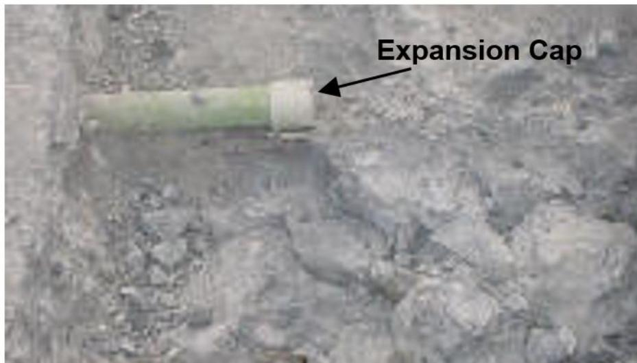
a. View of expansion cap on dowel bar
