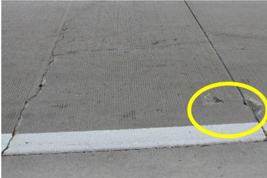
**g. Transverse cracking of UBCOC due to severely misaligned dowels, yellow oval shows the exposed end of a misaligned dowel**
