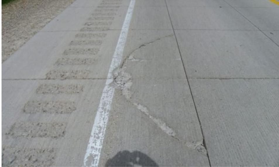
**c. Diagonal longitudinal crack over widened section**
