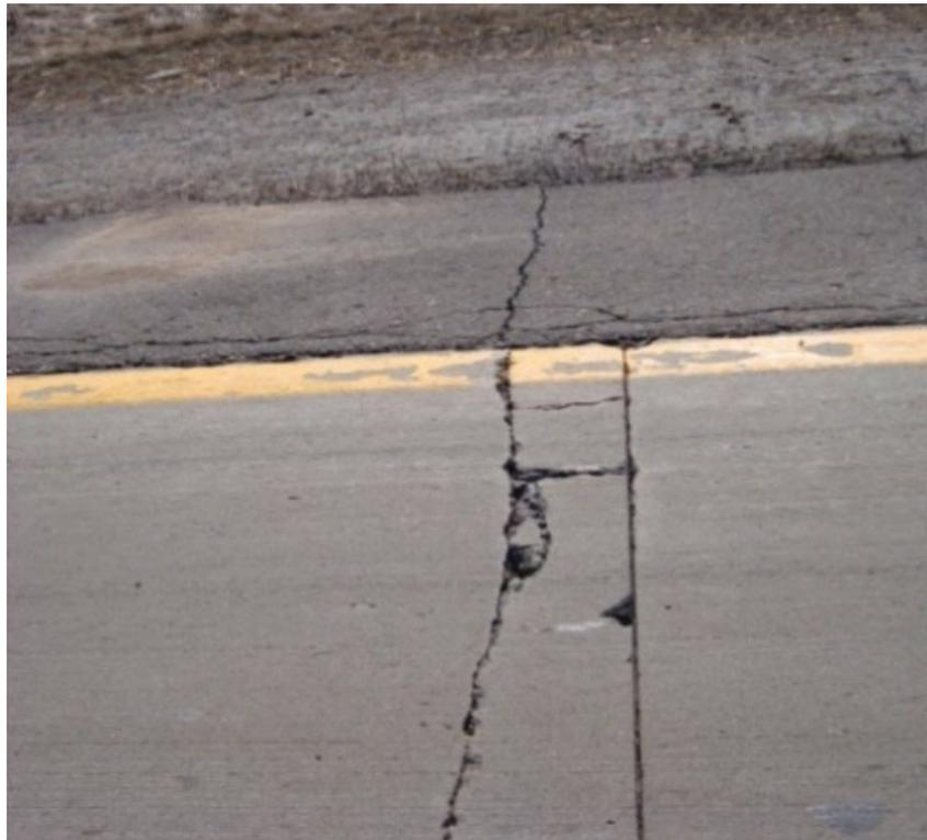
**e. Transverse reflection cracking**
