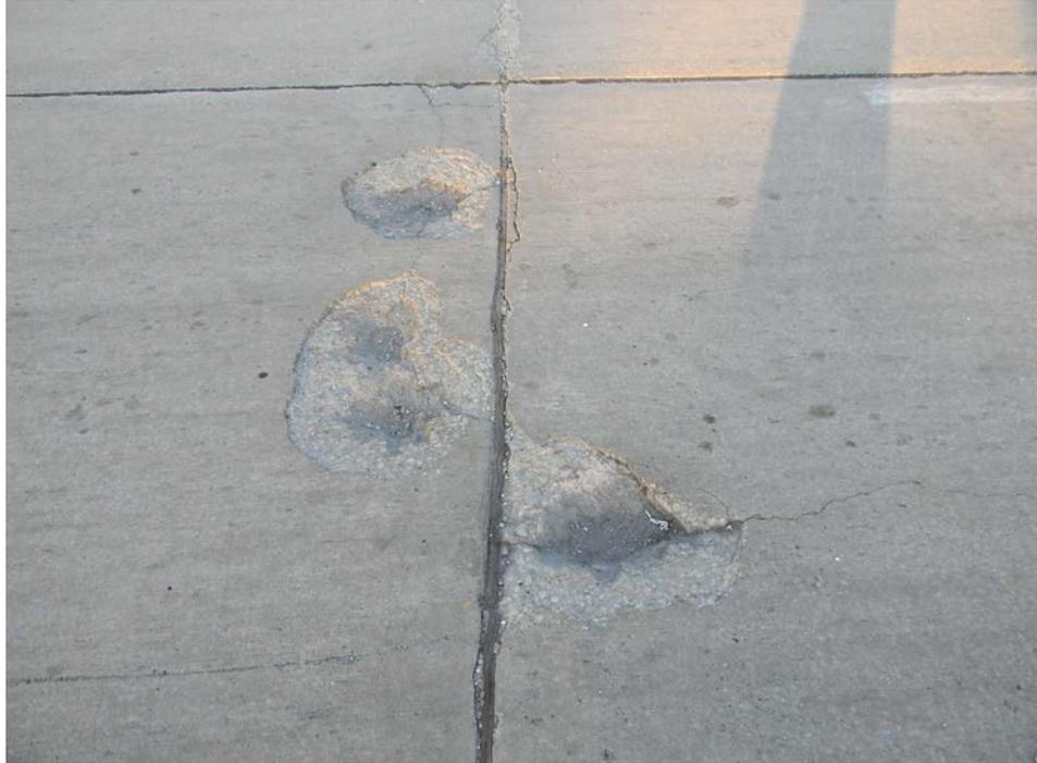
**b. View of an improper placement of an expansion cap on the end of a dowel bar resulting in expansive pressure on the concrete causing spalling**
