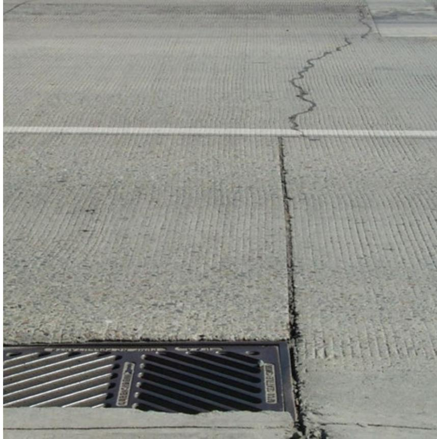
**b. Sympathy crack from joint aligning with catch basin**
