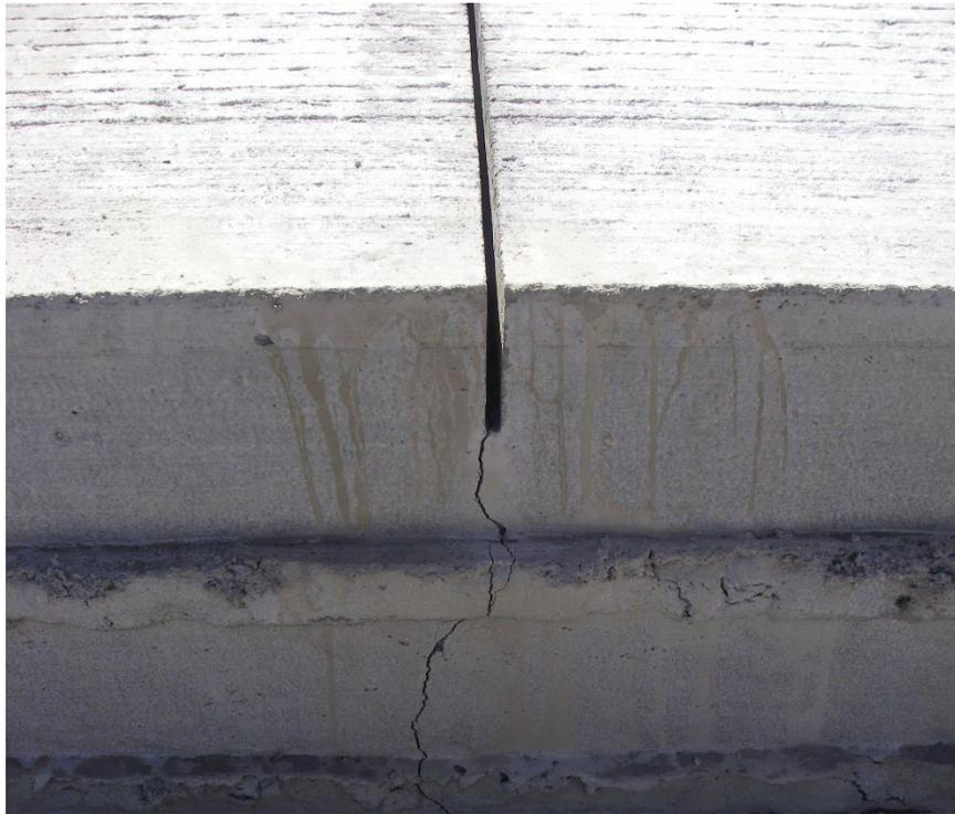
**a. Proper weakened plane saw cut and induced crack under the saw joint**
