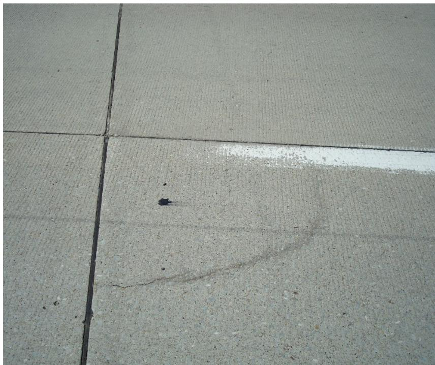
**a. Low-severity interior corner crack**
