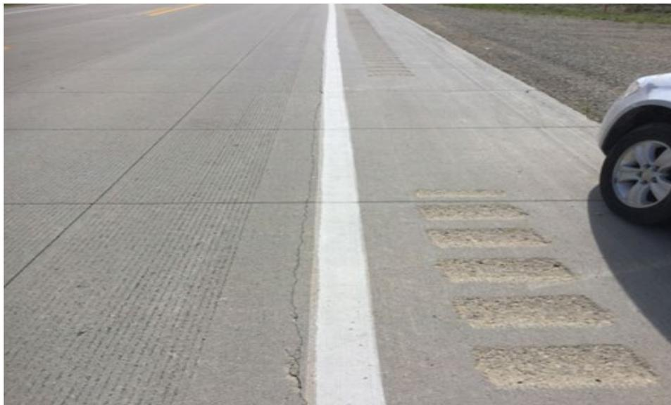
**d. Longitudinal crack over widened section**
