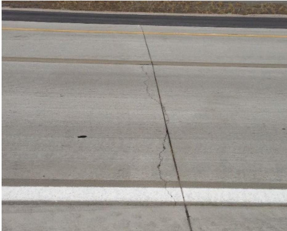
**g. Joint spalling, possibly due to late sawing or saw cut not directly over existing pavement joint/crack**
