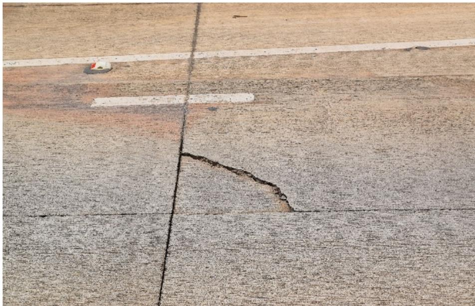
**d. Corner break and settlement due to subgrade soil movement under traffic**
