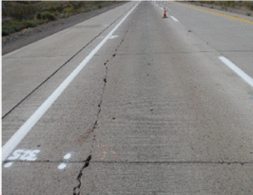
**b. Longitudinal crack in outer wheel path of the travel lane**
