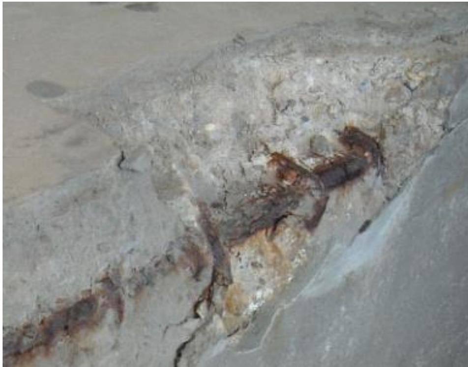
**b. Close-up view of corrosion of reinforcing steel causing spalling**
