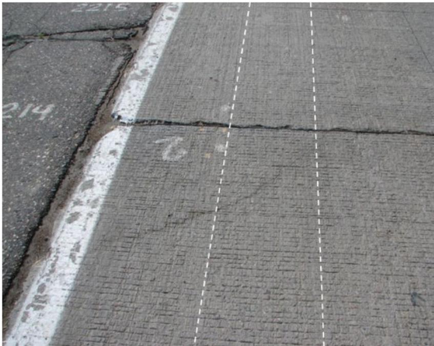
**c. Low-severity corner crack at exterior location with evidence of pumping along lane-shoulder joint**
