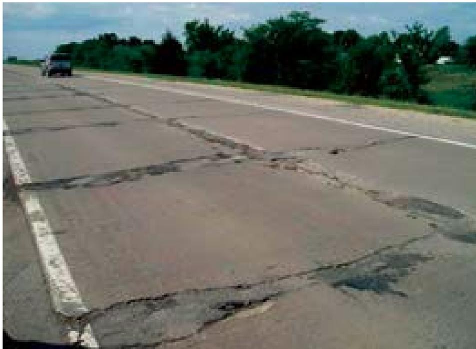
**a. Severe spalling on original concrete pavement (before overlay)**
