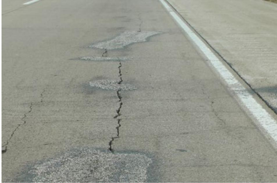
**c. High severity longitudinal cracking in CRCP**
