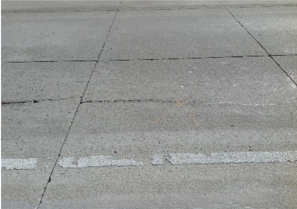
**a. Longitudinal cracking in the wheel path of UBCOC with tied shoulders and widened sections**
