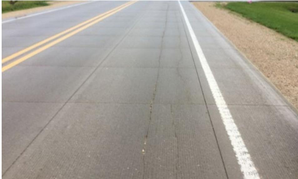
**a. Longitudinal cracking in the wheel path of a UBCOA with tied shoulders and widened sections**
