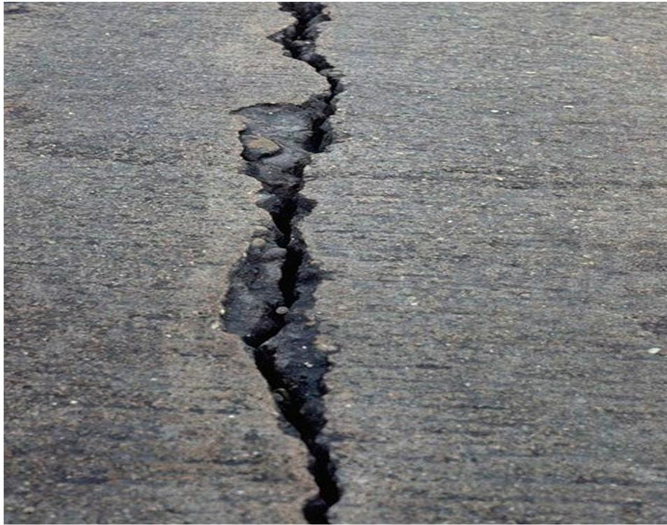
**a. High severity transverse cracking in CRCP**
