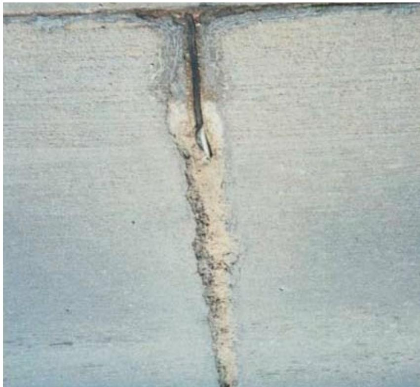
**b. Saturated joint backer rod damage**
