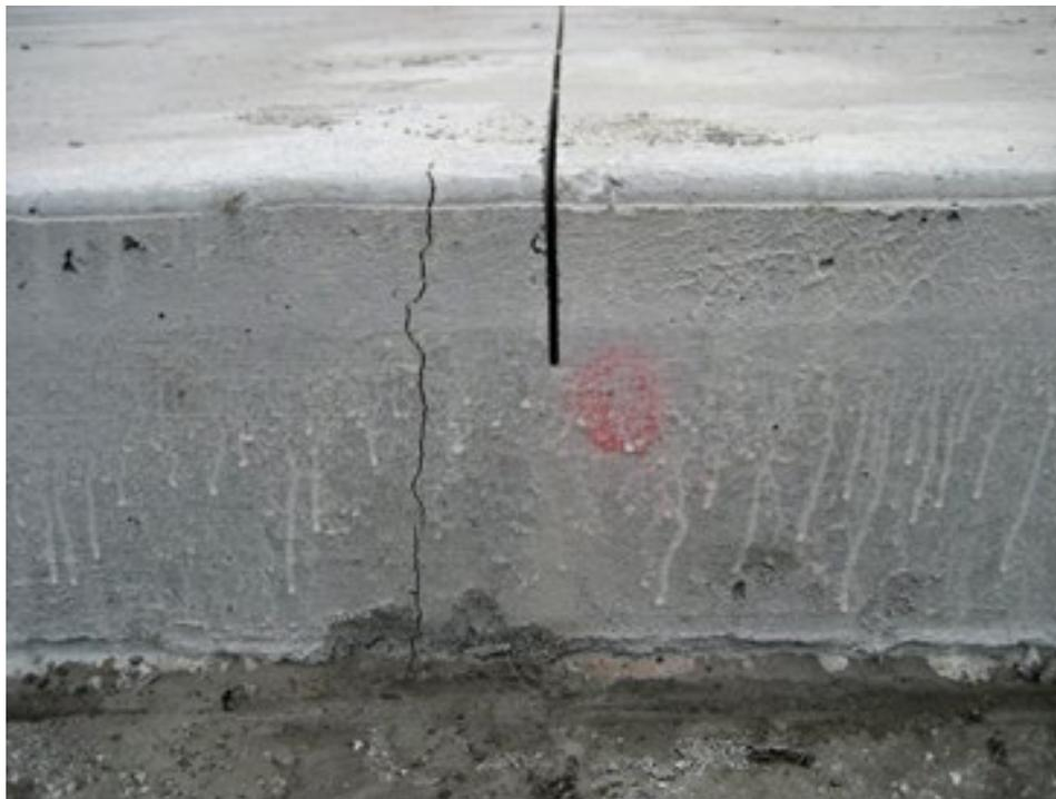
b. Slab cracking occurring parallel to weakened plane saw cut
