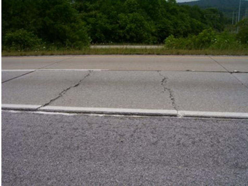
**b. Multiple transverse cracks on JPCP**
