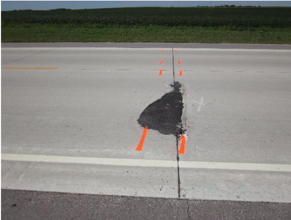
\*The patch and the orange pavement marking (from ground penetrating radar (GPR)) clearly shows the distress occurring where the dowel bar basket moved outside the joint proper.
