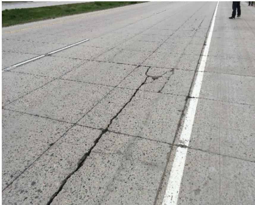
**i. Multiple longitudinal cracking in wheel paths**
