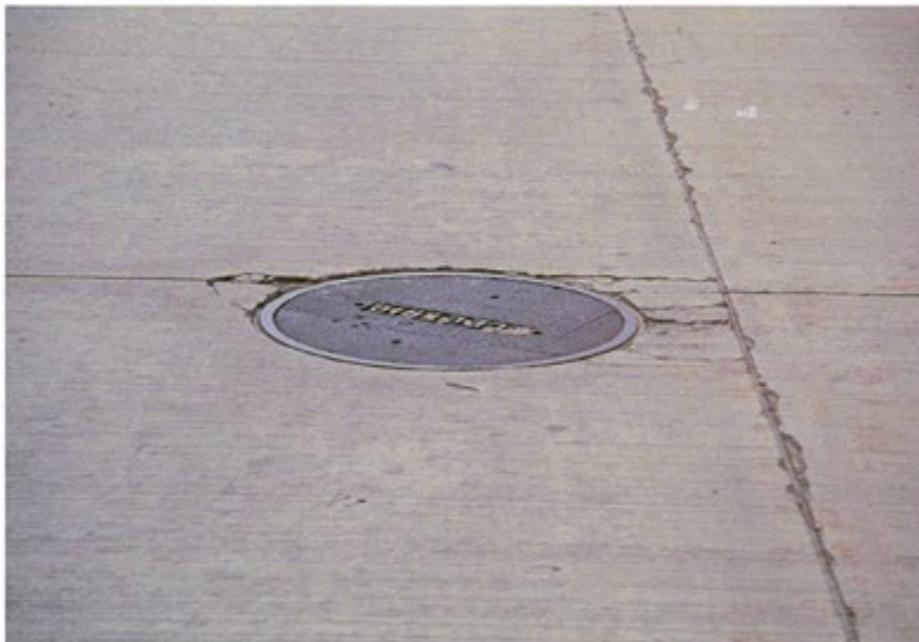
c. Cracking caused by lack of jointing to isolate a manhole
