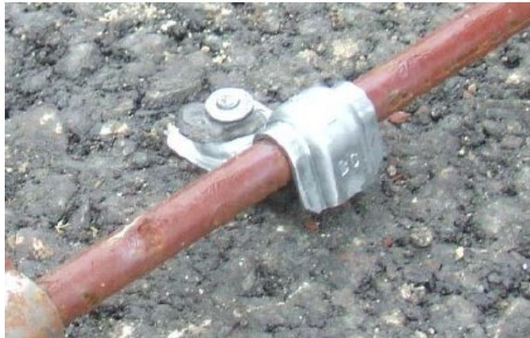
b. Anchor clip for dowel bar anchoring
