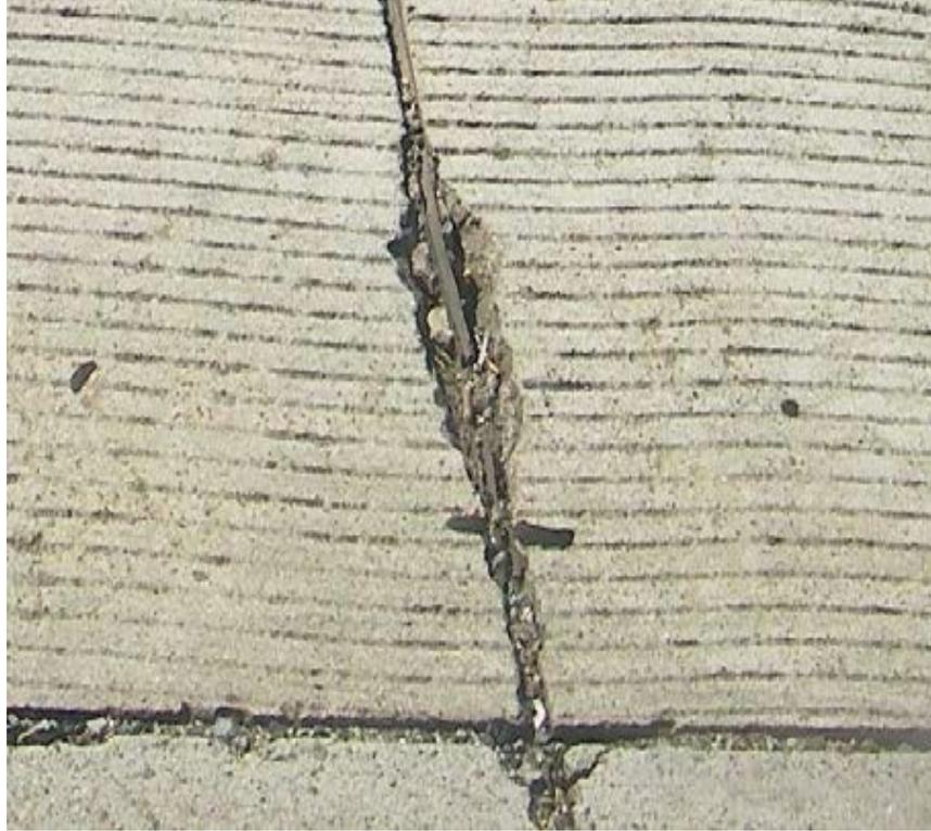
**d. Incompressible joint damage**
