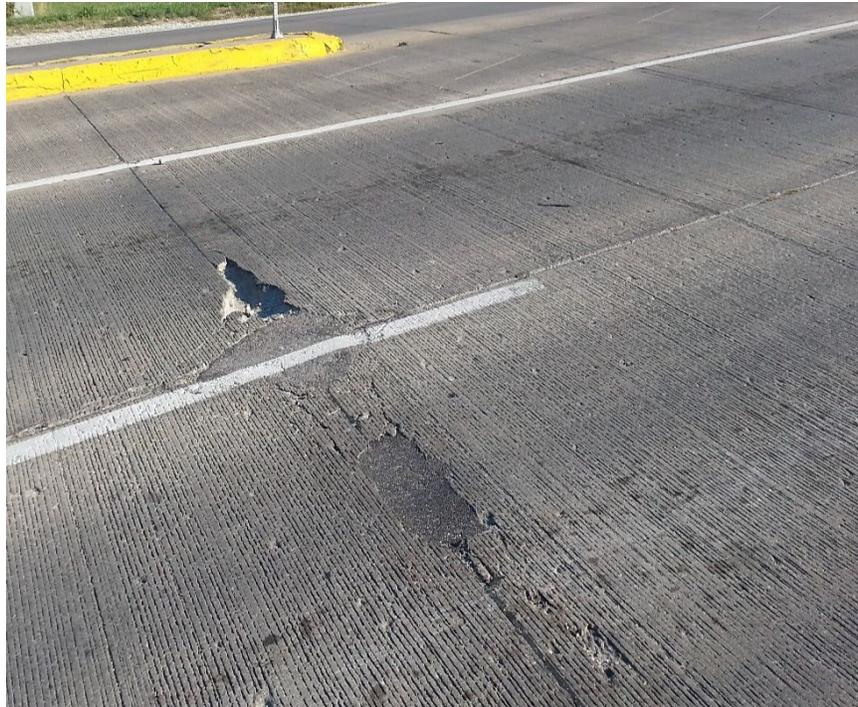
**e. Deflection spalling from heavy vertical loads**
