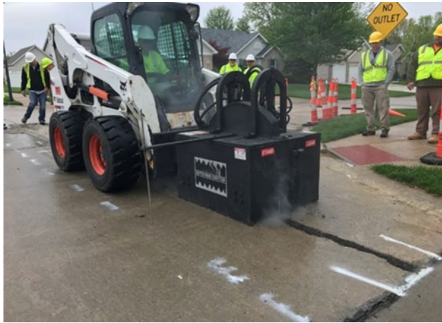
Figure B-19. Milling head attached to skid steer for concrete removal
