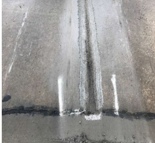
Figure B-20. Surface after milling and broom cleaning
