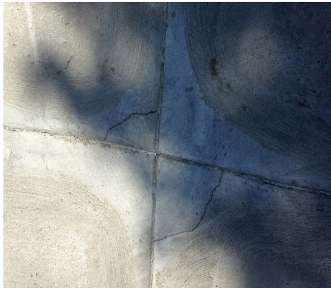
Figure B-22. Cracked PDR in intersection area
