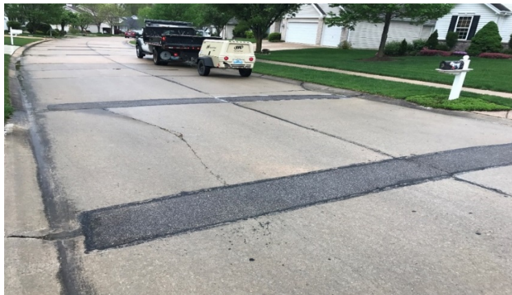
Figure B-18. 24-in. wide asphalt patch
