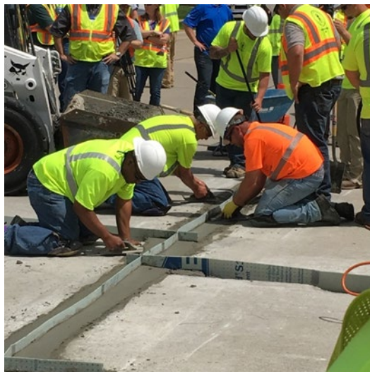
Figure B-21. Installing compression relief board
