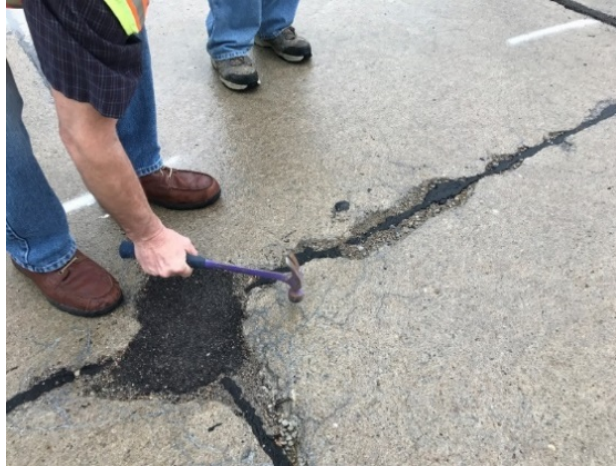
Figure B-17. Damage appearing as spider-like cracks around the joint area
