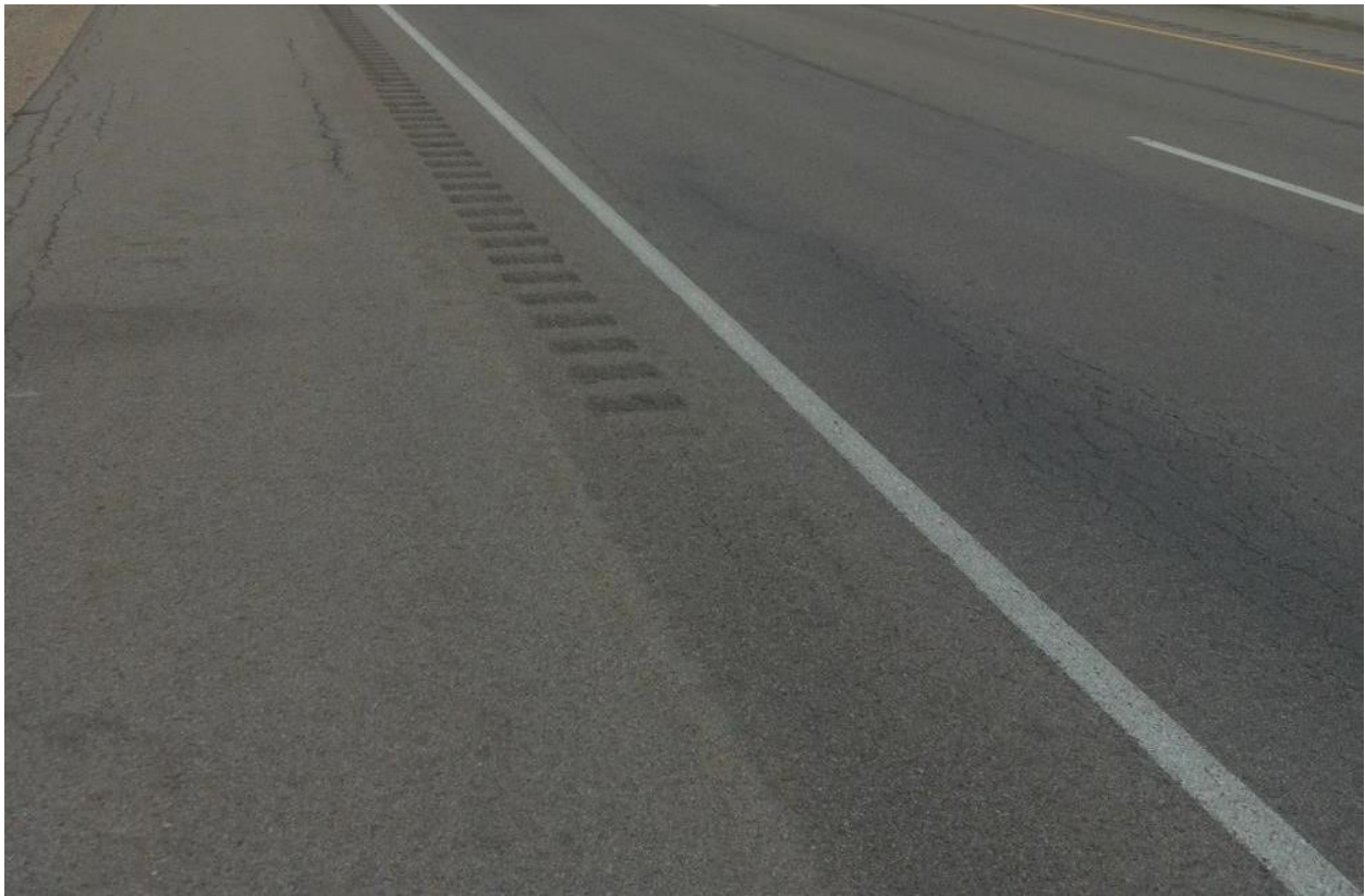
Figure C-7. Rutting and fatigue cracking on I-80
