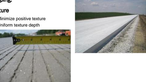
The image shows two views of a concrete surface. On the left, a close-up of a textured surface with a yellow measuring tape. On the right, a long view of a concrete slab with a curing compound being applied.
