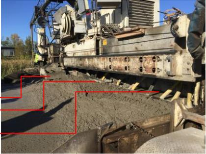
The image shows the front of a paver with concrete being laid. Red arrows point to specific components: 'plow', 'metering gate/strikeoff', and 'head in grout box'.
