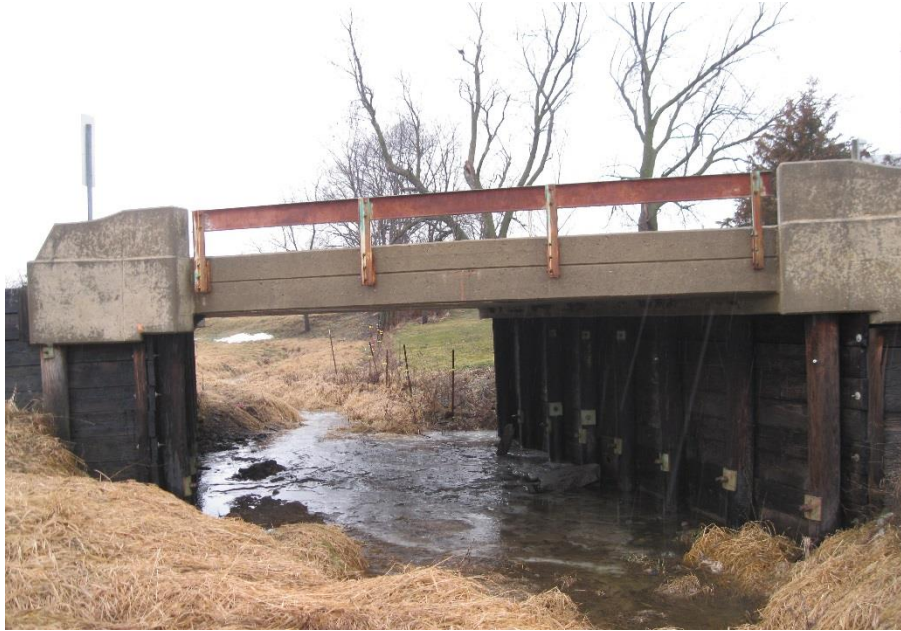
Figure 3. Johnson County Bridge elevation view
