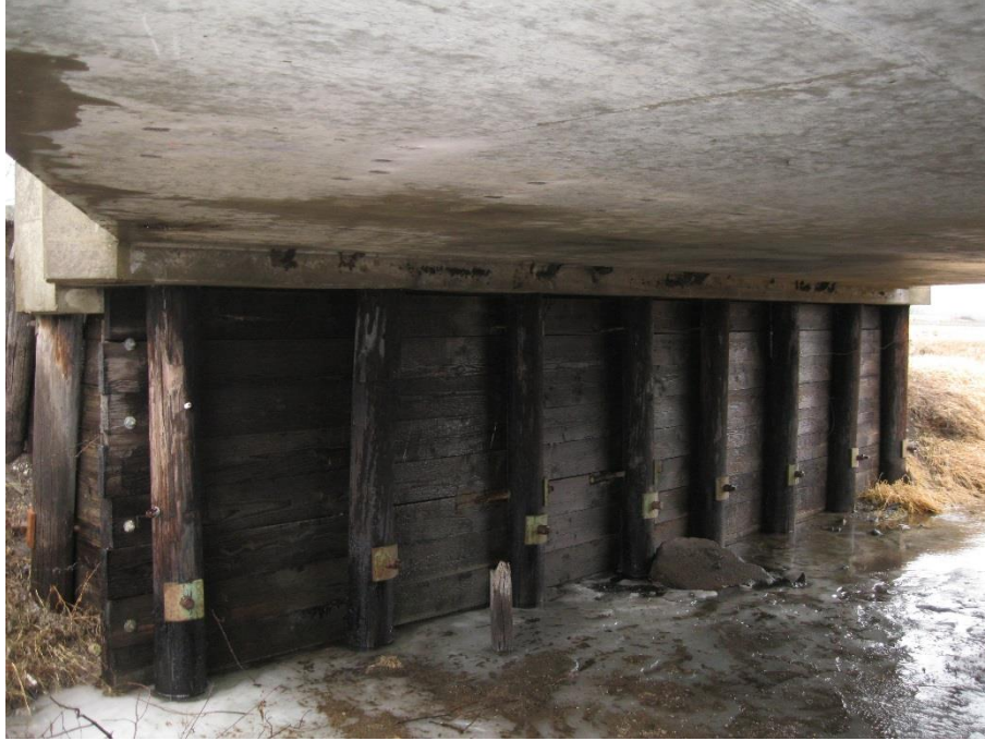
Figure 5. Johnson County Bridge bearing
