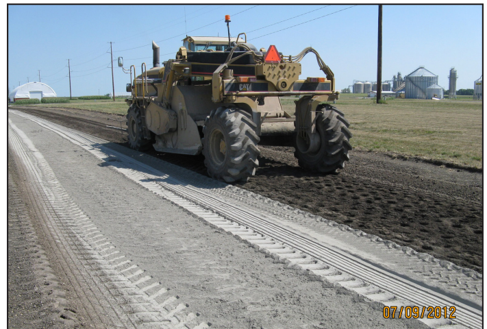
Figure 4. Mixing of subbase with PC on 7th St. North
