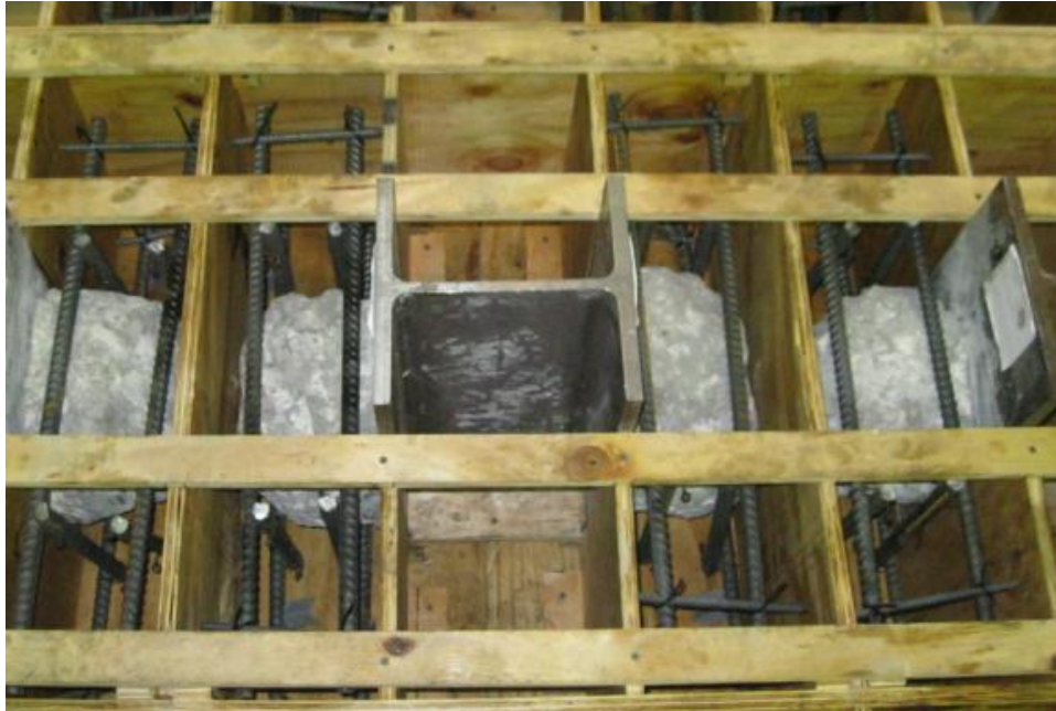
Figure 43. Specimens, reinforcing steel, and formwork (Dang 2013)
