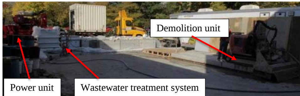
Figure 8. Hydrodemolition site (Dang 2013)
