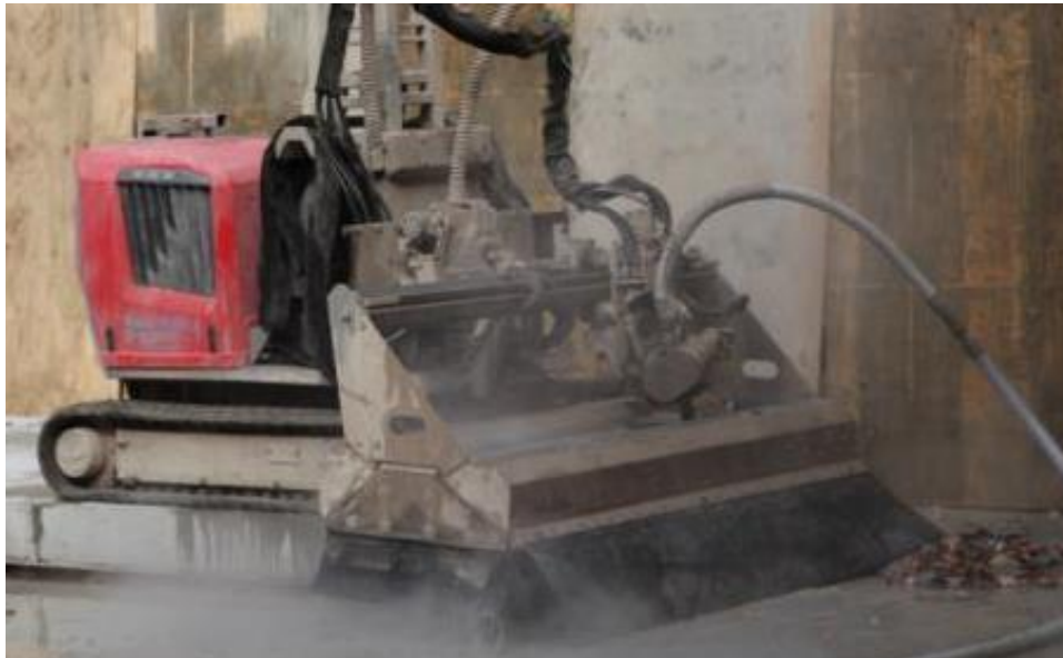
Figure 9. Hydrodemolition trial (Dang 2013)
