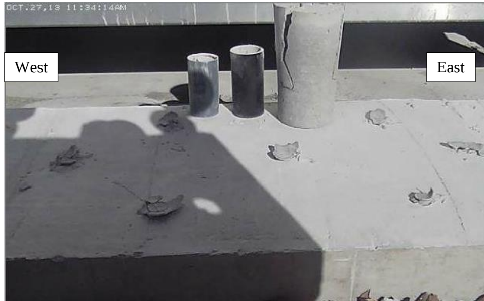
Figure 19. Chemical splitting on day two (after 48 hours)
