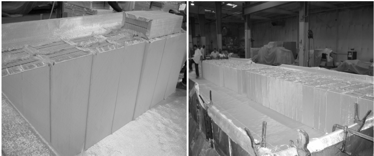
Figure 5. Installation of FRP wrapped foam bottles
