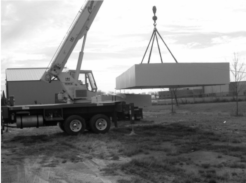
Figure 11. Unloading of individual deck panels
