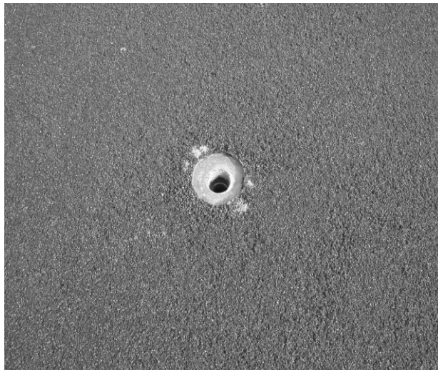
Figure 8. Threaded insert for installation of lifting lugs
