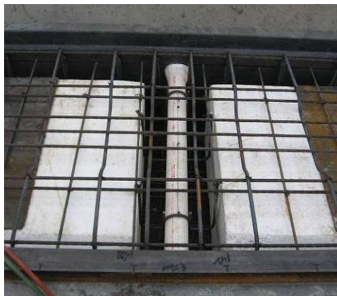
Figure 2.10. Photograph of midspan transverse tie duct
