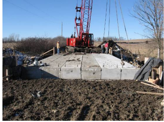
d. box girders in final position
