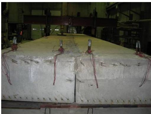
c. girders with the shear key cast.
