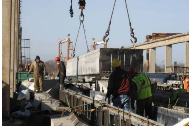
Figure 2.11. Photograph of crew lifting girder out of forms
