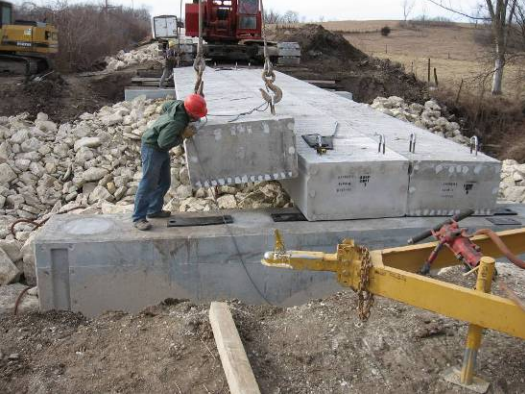
c. placing girder into final position
