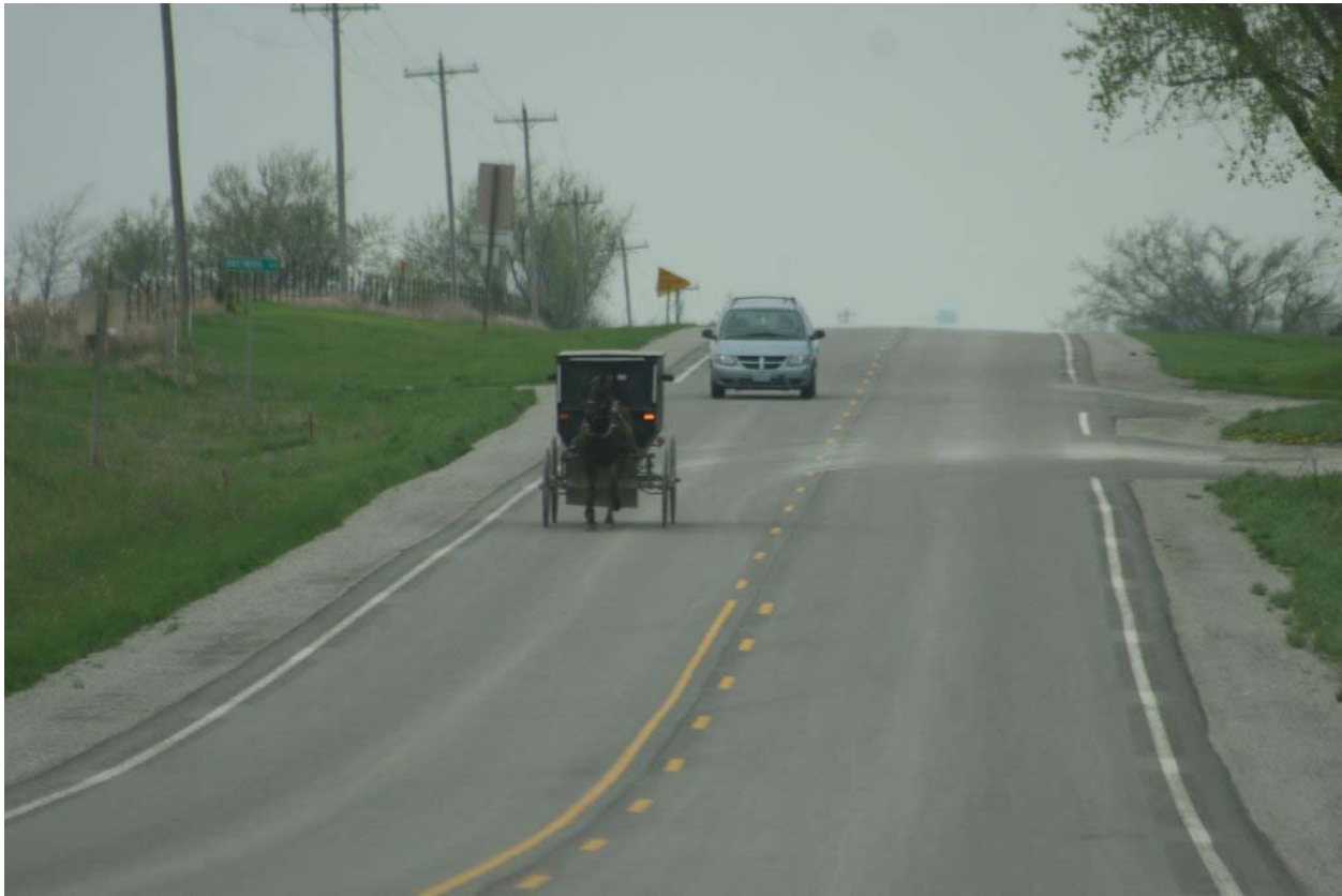
Figure 5-21. Edge line rumble stripes in place along Iowa 2 (image courtesy of Neal Hawkins, CTRE)
