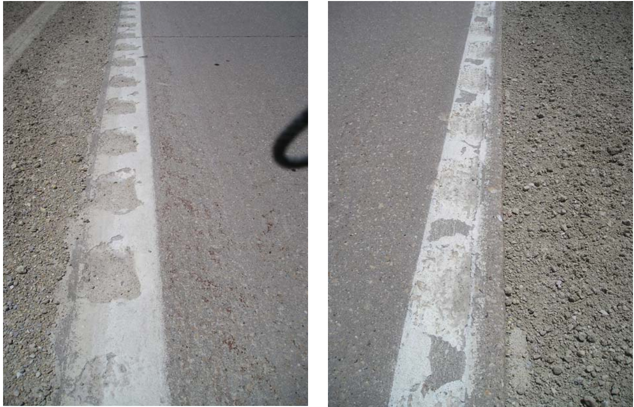
Figure 5-13. W-13 pavement markings in spring and after wear over winter, showing more wear in the groove than in the flat section
