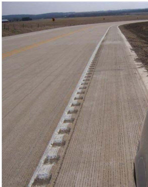
Figure 4-18. Rumble stripe installation on E-16
