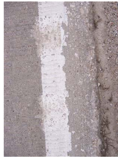
Figure 5-15. Similar wear for rumble stripe and flat section (taken spring 2009). F-29 is on the left and P-53 is on the right.
