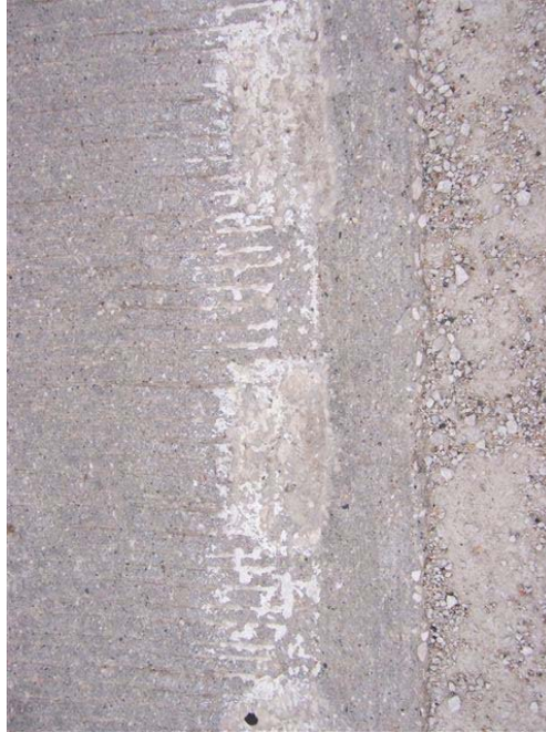
Figure 5-18. Another portion of P-53 showing less wear in the rumble stripe than in the flat area (taken spring 2009)
