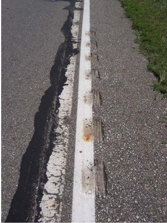
Figure 3-14. Photos showing difficulty in maintaining painted edge line alignment within rumble stripe installation
