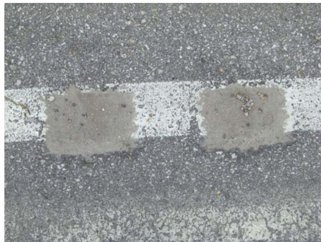
Figure 5-3. Rumble stripe with caked fines in bottom
