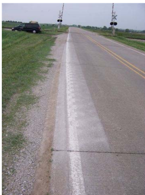
Figure 4-6. Rumble stripe installation on P-53
