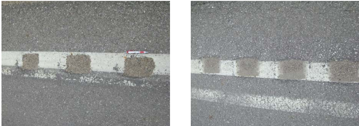
Figure 5-2. Rumble stripes filled with sand
