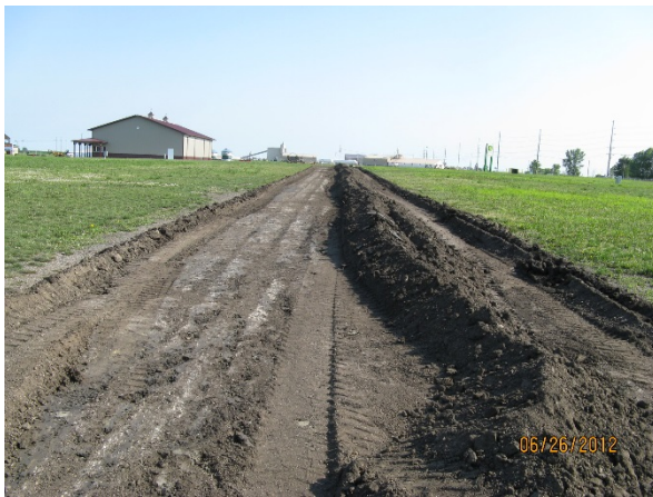
Figure 79. Pavement foundation profiles with (a) 4 in. geocells on 3rd St. North, and (b) 6 in. geocells on 3rd St. South
