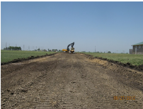
Figure 80. Removal of existing granular subbase on 3rd St.
