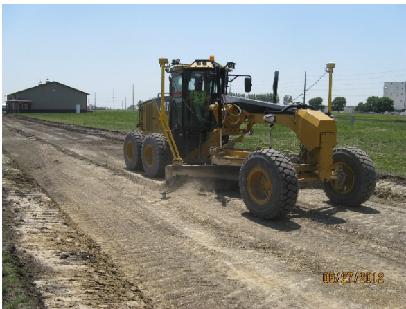
Figure 80. Removal of existing granular subbase on 3rd St.
