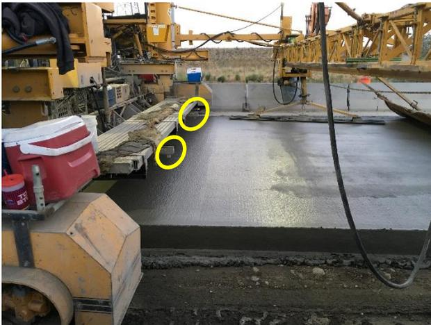
Figure 1. RTP (yellow ovals) Installed Behind the Dowel-Bar-Inserter (with OCB).
