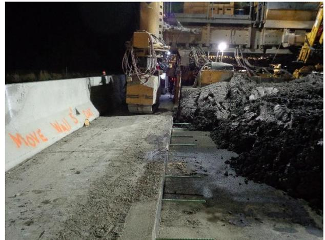
Figure 2. Concrete Dumped Directly in Front of the Paver and Right Side of Paver Matching Existing Slab.
