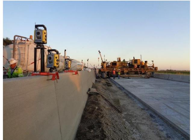
Figure 4. Trimble Stringless Robotic Lasers Setup on Median Barrier
