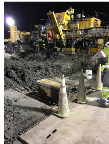
Figure 4. Paving at a Drainage Structure
