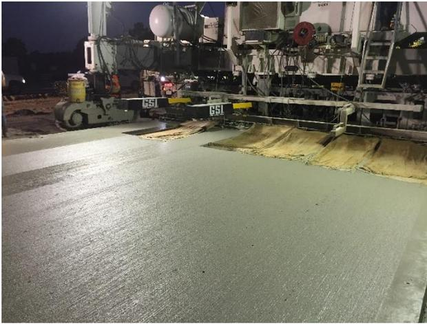
*Figure 1. Gomaco GSI Mounted to G-Z S-850 Paver With a Float Pan*
