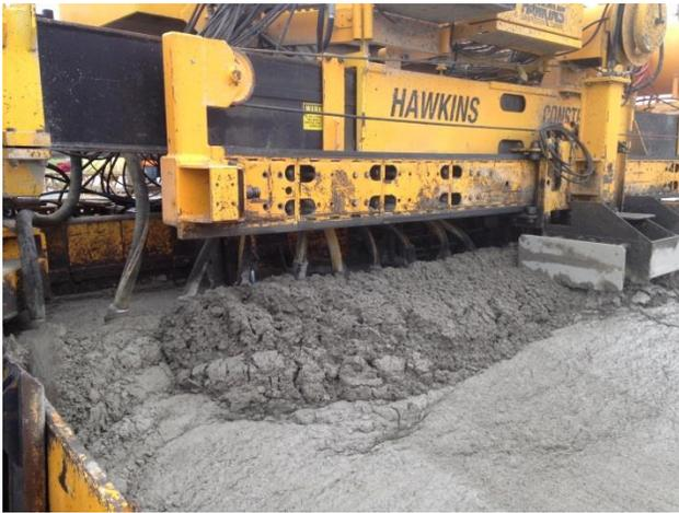
*Figure 3. Concrete at the Front of the Paver (relatively high head pressure)*
