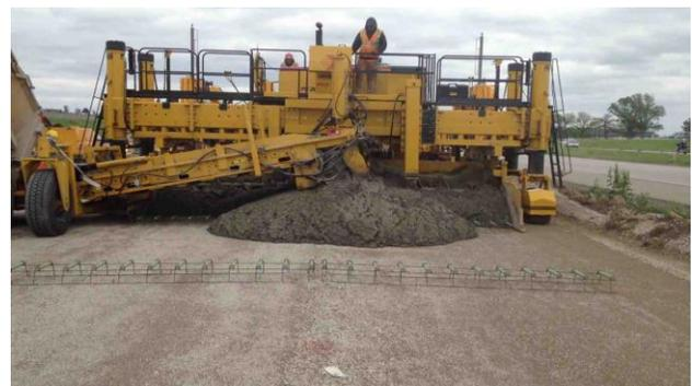
*Figure 2. Concrete Deposited on Dowel Baskets Ahead of the Paver*
