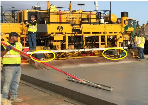
*Figure 1. Ames RTP Mounted to Gomaco 2800 paver with DBI (yellow ovals, note that GSI sensors are mounted adjacent to the RTP).*
